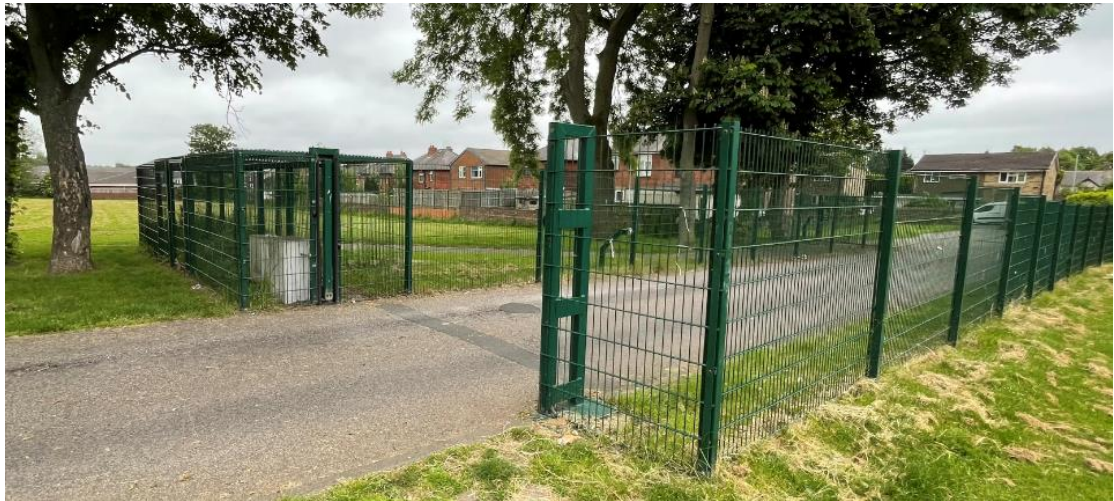
Photo 11 – Weld mesh grid type fencing to perimeter of vehicular entrance of Old Bank Road.
