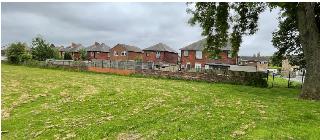
Photo 12 - Lack of perimeter security to properties at South of site.
