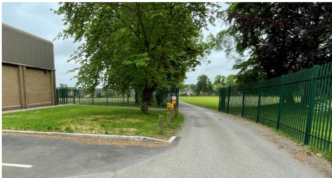
Photo 4 – Security fencing to main vehicle access road and school car park.
