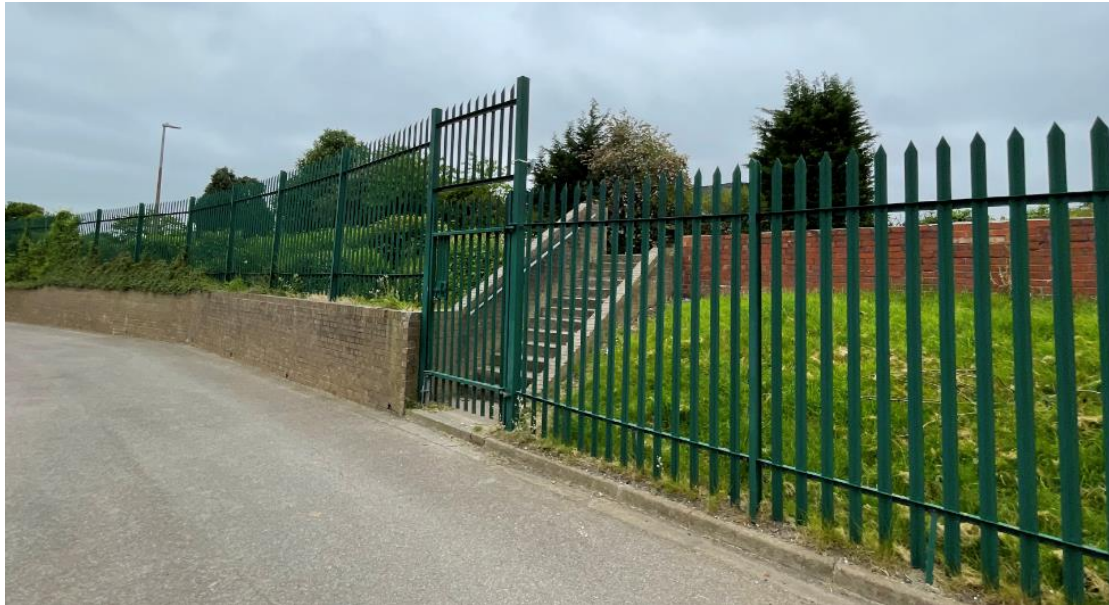
Photo 3 – Security fencing and pedestrian gate to North boundary of site and housing estate off Moor Park Lane.
