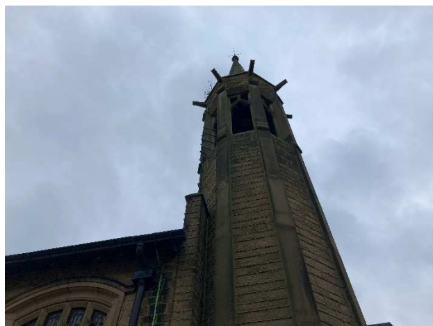
Photo 14: The belltower on the northern aspect, viewed from the east.
