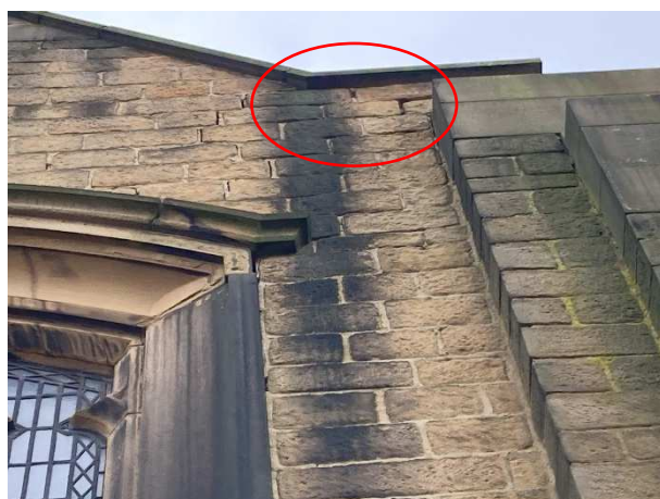
Photo 8: Missing mortar on the eastern aspect, viewed from the east.
