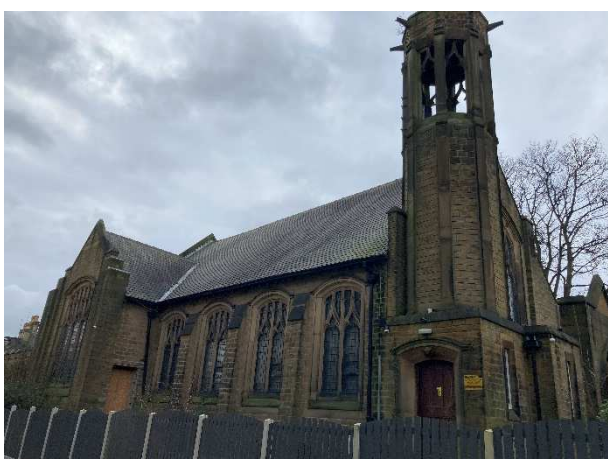
Photo 5: The building on site, viewed from the northeast.
