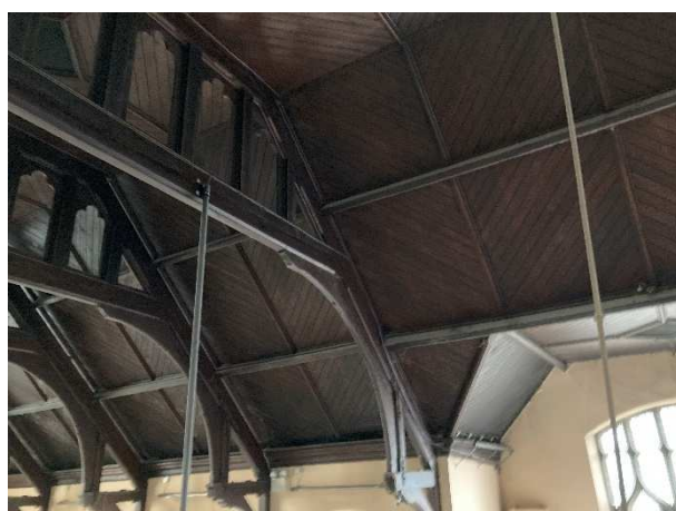
Photo 6: Wooden sarking and hammer beam trusses supporting the roof.
