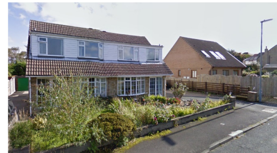
Nearby residential development – Denby Park Drive
