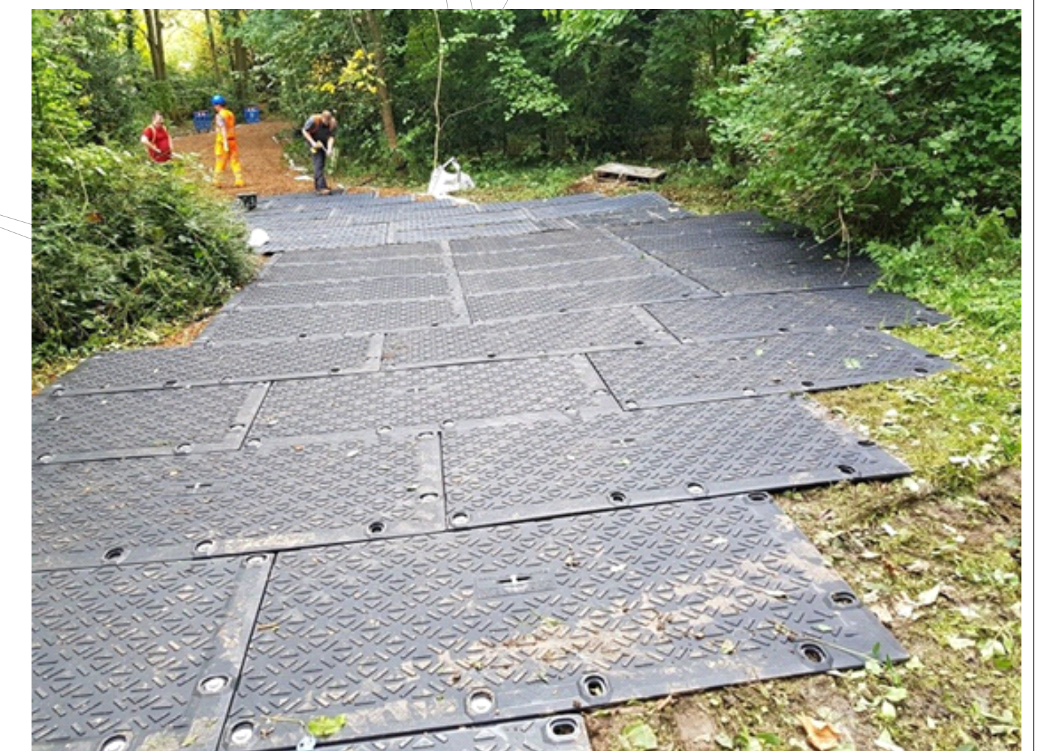
Inset 2: Ground Protection Boards
