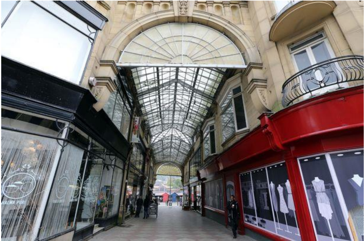
Figure 5 – Existing shopfront to Northgate/Kingsway Arcade looking towards the market place
