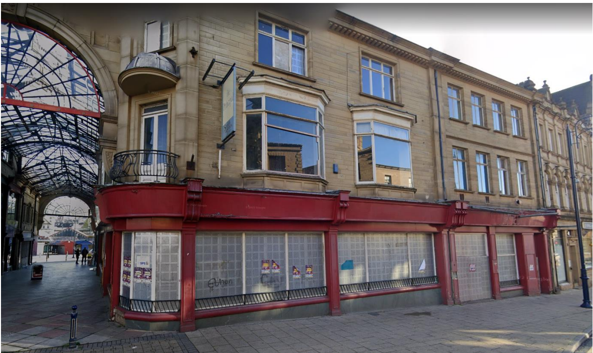
Figure 2- Existing shopfronts to Northgate
