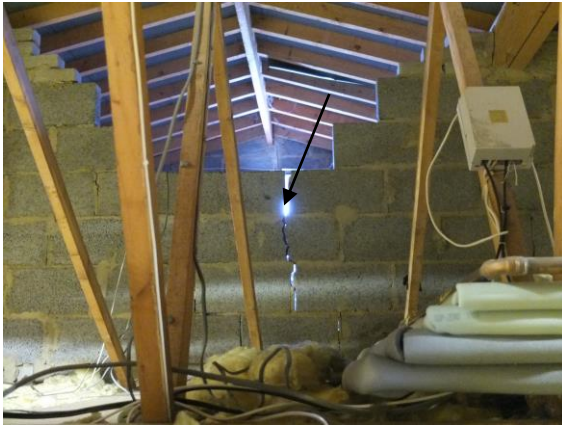
Internal separation of blockwork in central area to attic space
