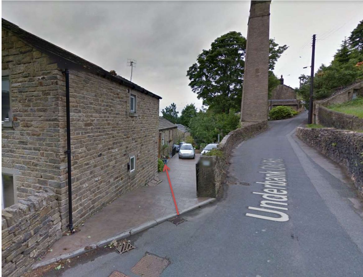
Street View of the Site from the entrance to 110 Underbank Old Road.
