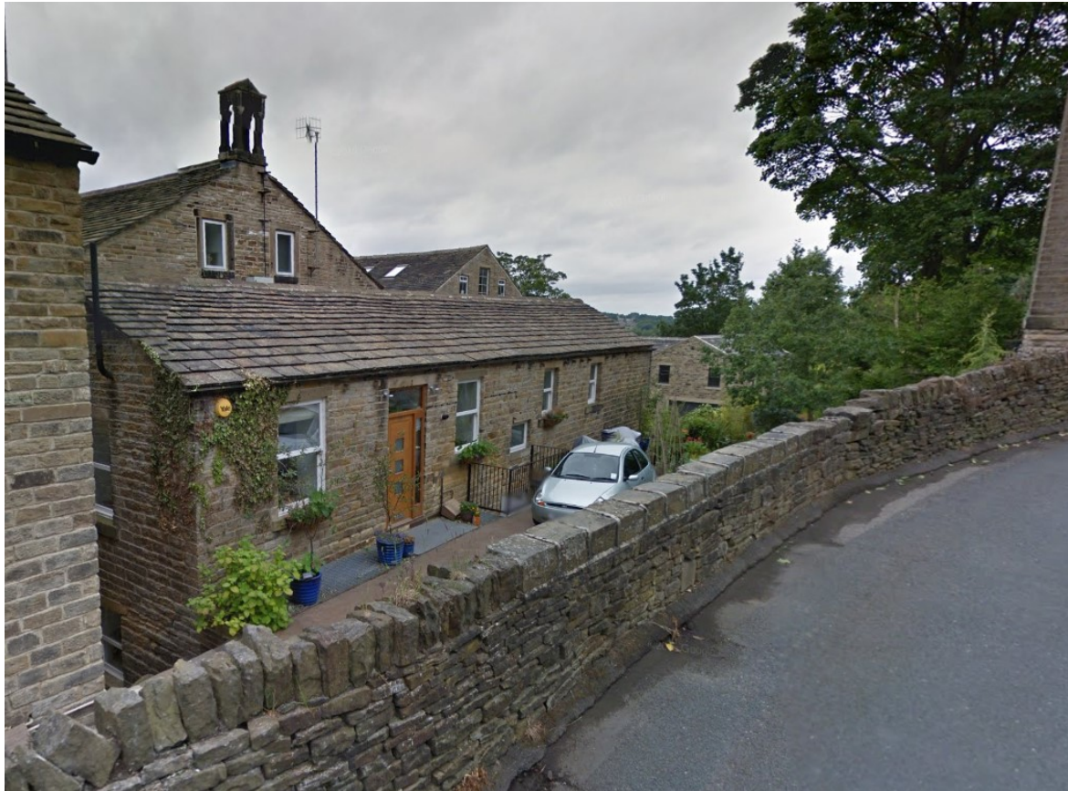
Street View of the Site from Underbank Old Road.
