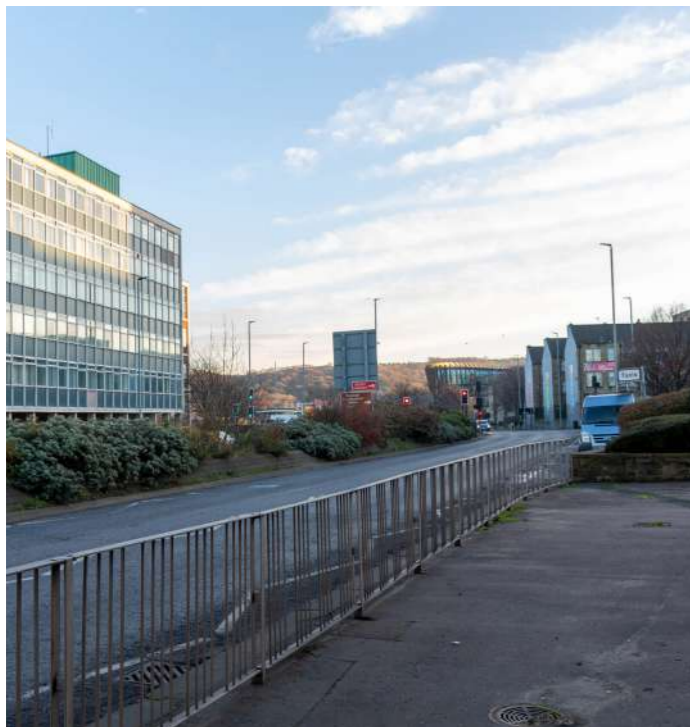
View south towards University campus
