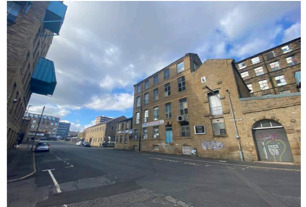
2. View north west down Quay St
