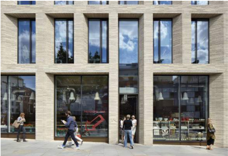
Turnmill Building - London
