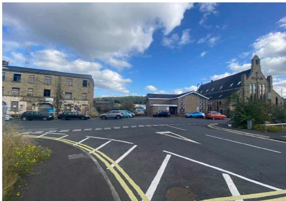
9. View west from the junction of Pine St and Old Leeds Rd
