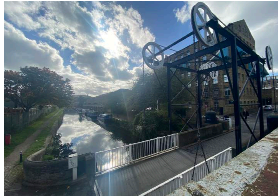
1. Canal bridge over the Broad Canal
