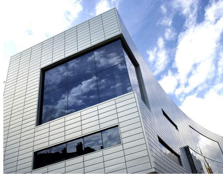
Richard Steinitz Building - University of Huddersfield
