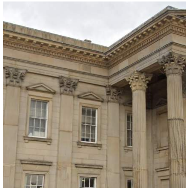
2. Huddersfield Railway Station
