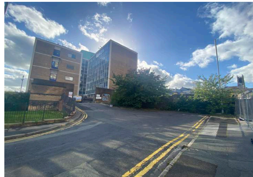
7. View south towards BT openreach building
