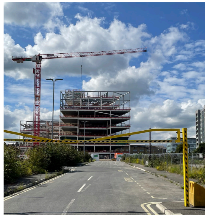
Current Site Condition
