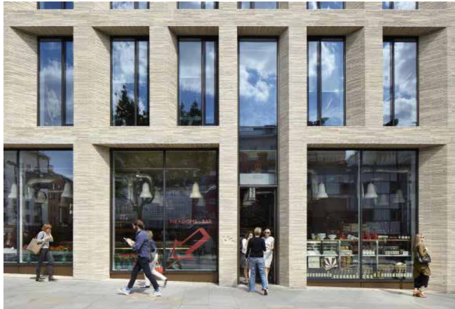
Turnmill Building - London
