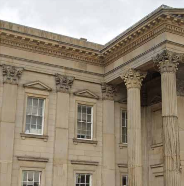
2. Huddersfield Railway Station
