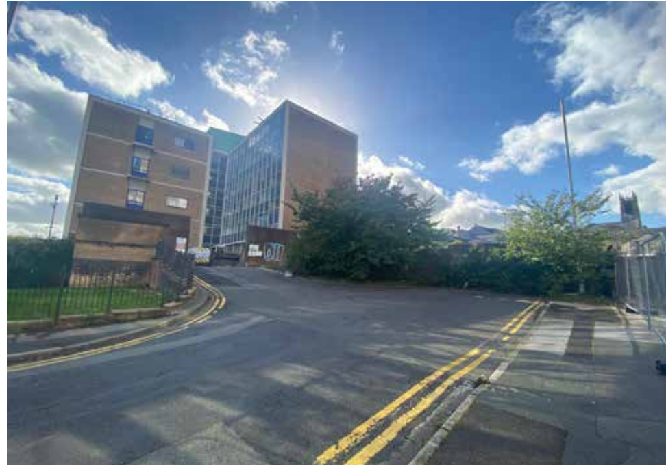
7. View south towards BT openreach building
