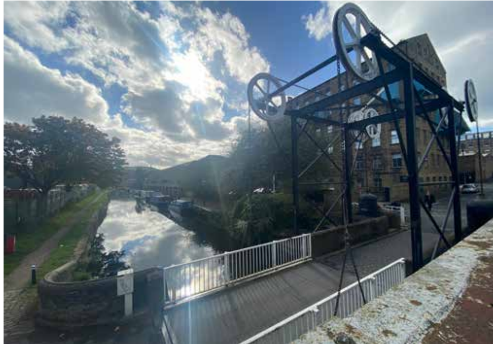
1. Canal bridge over the Broad Canal
