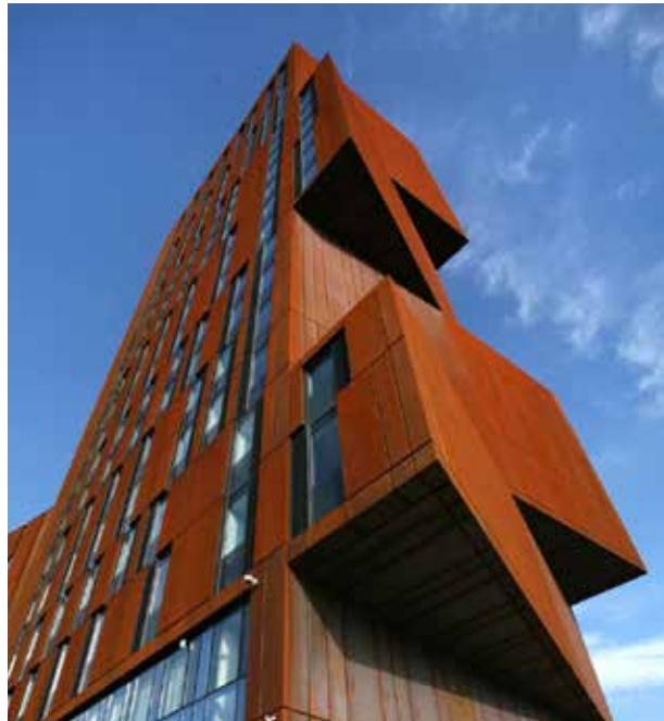
Broadcasting Place - Leeds
