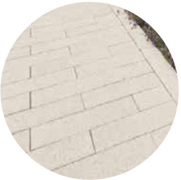
Silver grey pre-cast concrete slabs
