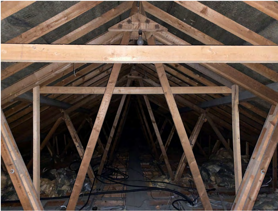
Photo 7. Interior of loft space in on-site building (Jan 2023)
