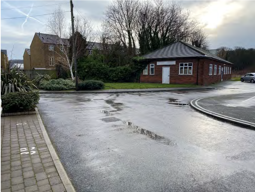
Photo 3. Looking south-east towards building in eastern part of the site (Jan 2023)
