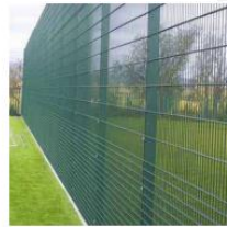
3.0m Rebound Weld Mesh Fencing to MUGA
