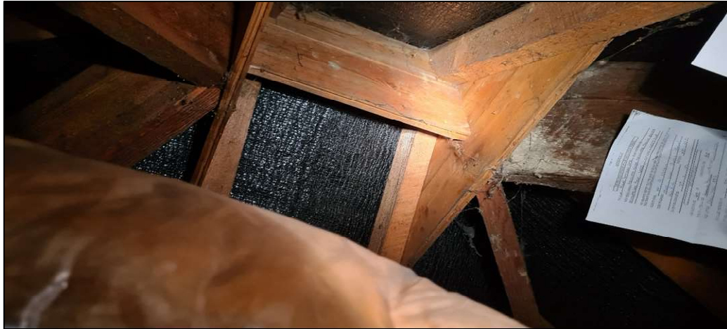
Building description - garage
