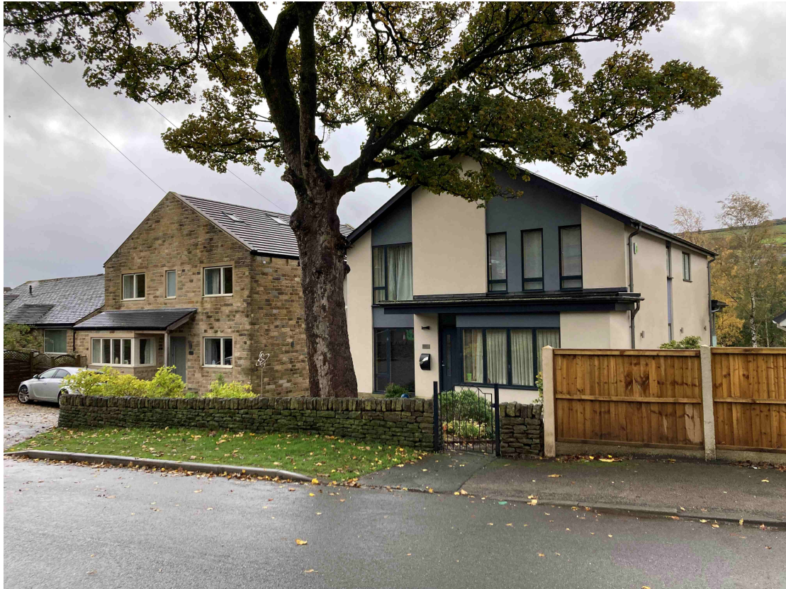
Photograph 3 - Recently Constructed Properties, 25 and 27 Burnlee Road
