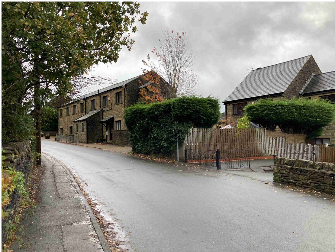
Photograph 5 - Two Storey Dwellings to the East of the Site, with the Neighbouring Property (Off Victoria Springs) to the Right of the Photograph.
