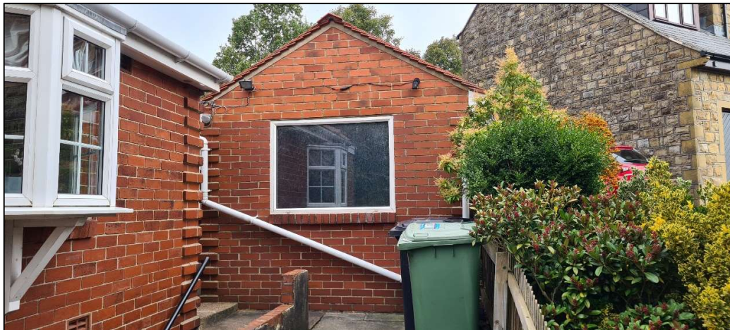
External inspection - garage
