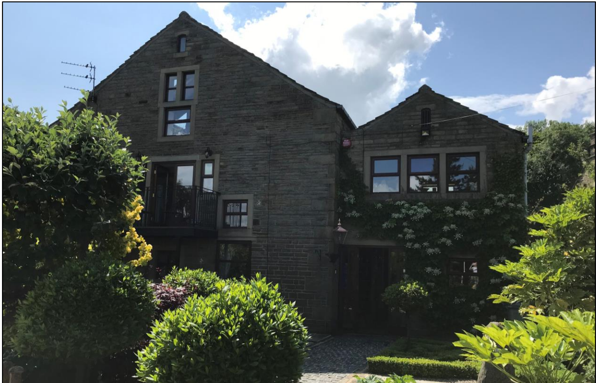
The front elevation of No. 159A Lane Head Road
