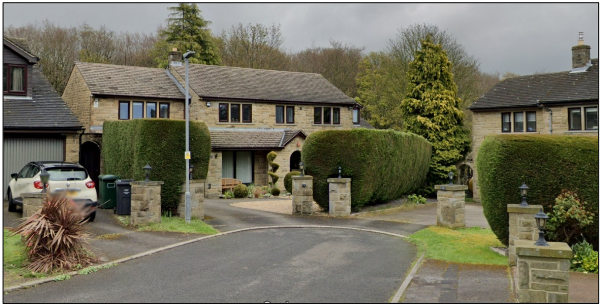
Front view of 18 St. Francis Gardens (No. 20 just visible to the left and no. 16 to the right)
