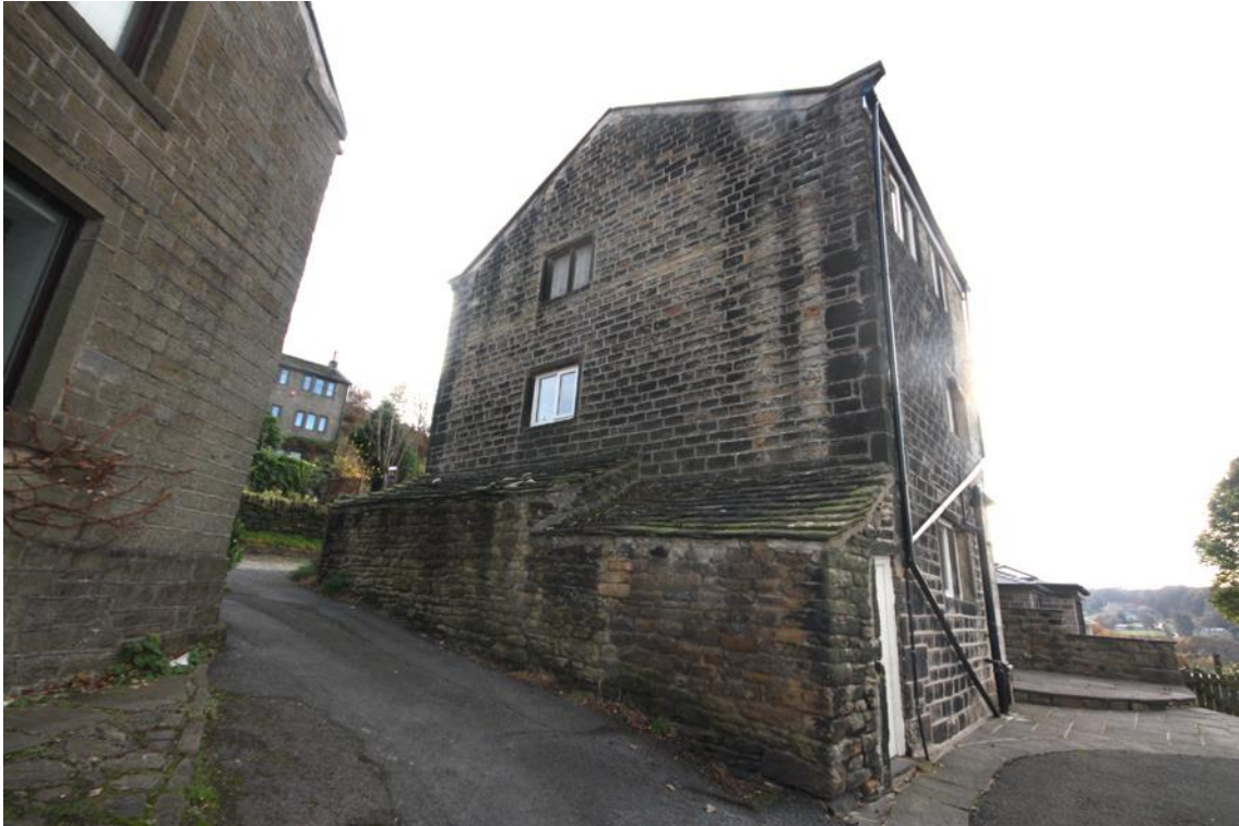
Fig.2 Photograph of the side elevation of No.59 Cliff Road
