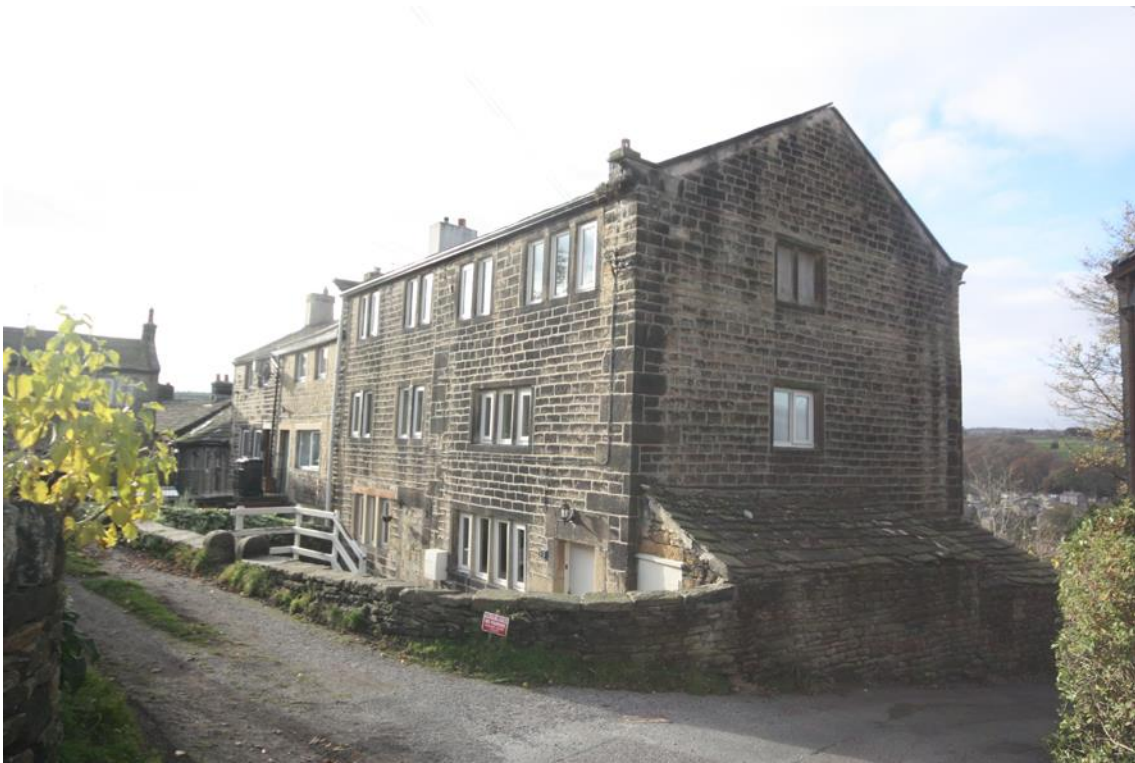
Fig.1 Photograph of the front and side elevation of No.57 - 59 Cliff Road
