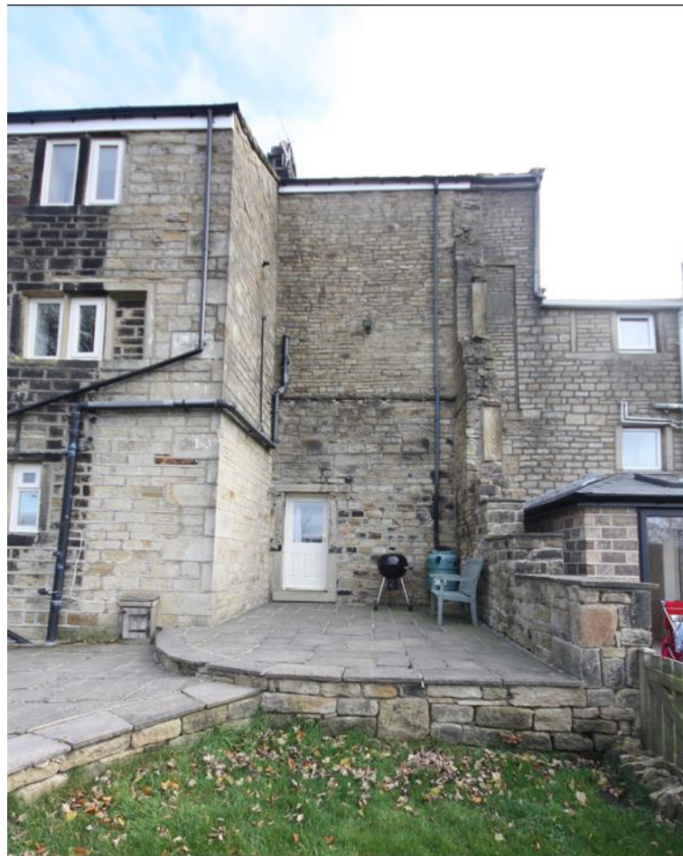
Fig.3 Photograph of the rear elevation of No.57 Cliff Road
