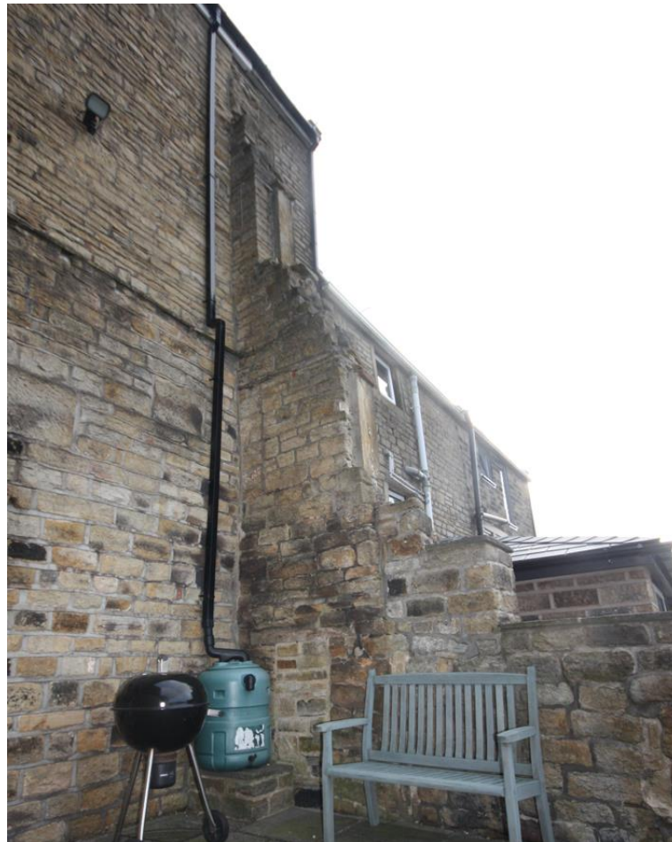
Fig.4 Photograph of external wall remains of building to rear of No.57 Cliff Road
