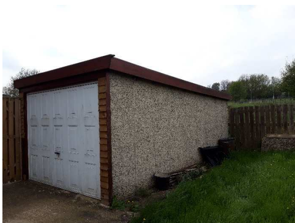
Photo 3: Garage present in the south west of the site which will be demolished.
