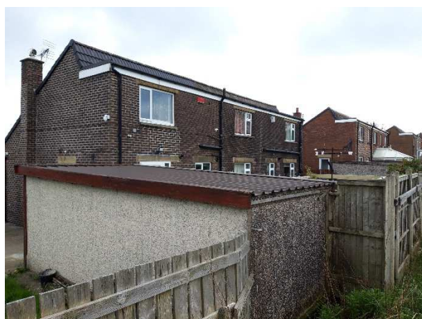
Photo 4: Rear view of the garage
