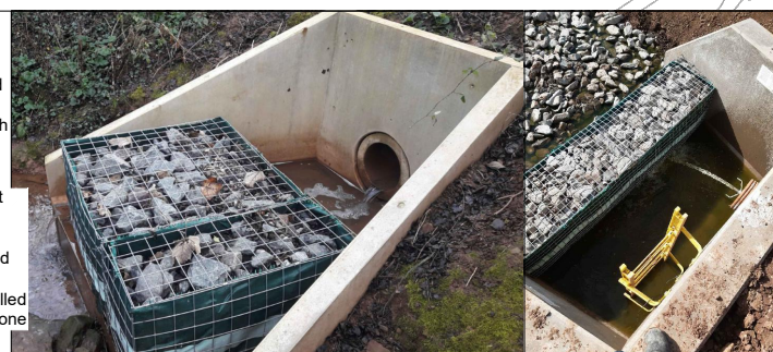
5 Inflow / outfall headwall gabion basket detail
