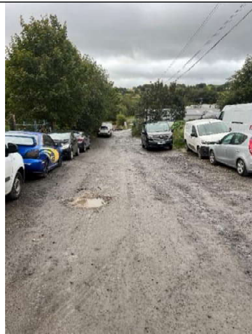
Photo 14 – Severely deteriorated surface, pooling of water in some areas.
