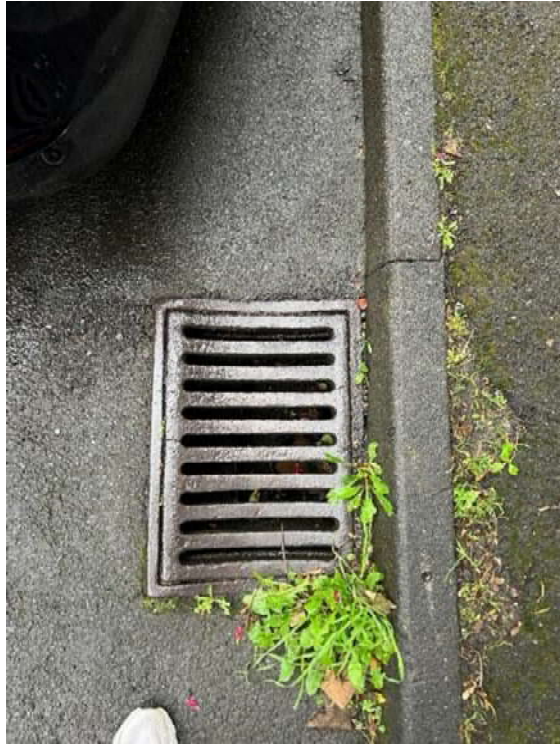
Photo 17 – Gully at bottom of Taylor Street clear
