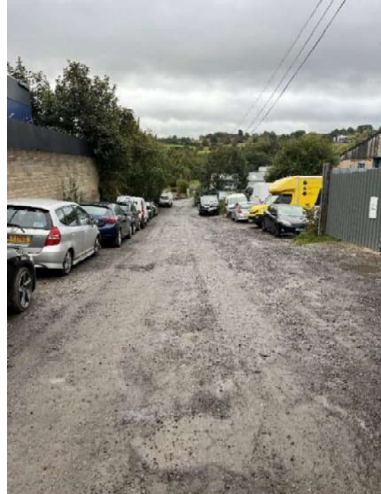
Photo 14 – Severely deteriorated surface, pooling of water in some areas.
