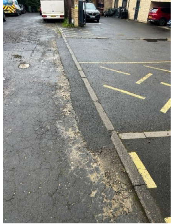
Photo 12 – Ramp has been installed for access
