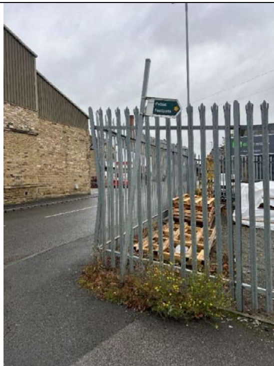
Photo 3 – kerbing not level and cracked, surfacing is fatigued and is pooling of water at far end of junction with Westgate
