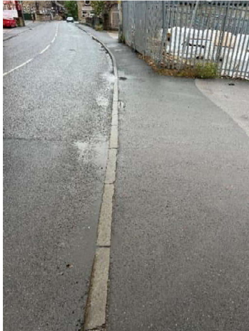
Photo 3 – kerbing not level and cracked, surfacing is fatigued and is pooling of water at far end of junction with Westgate
