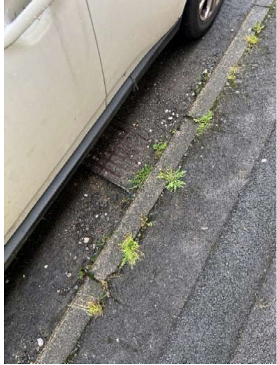
Photo 14 – Gully blocked
