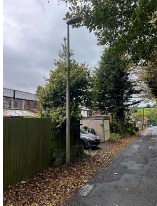
Photo 16 – Lighting column in acceptable condition
