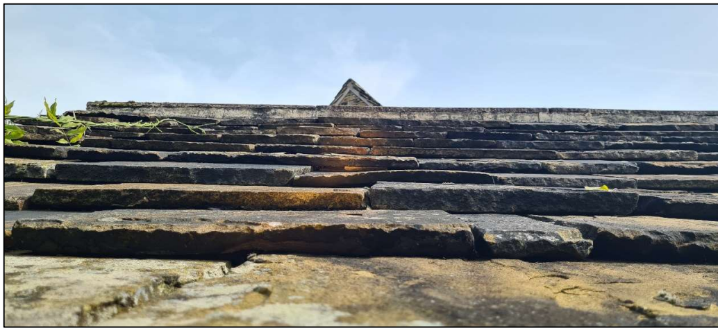
Plate 3. Gaps between the stone slates at the northern gable end.
