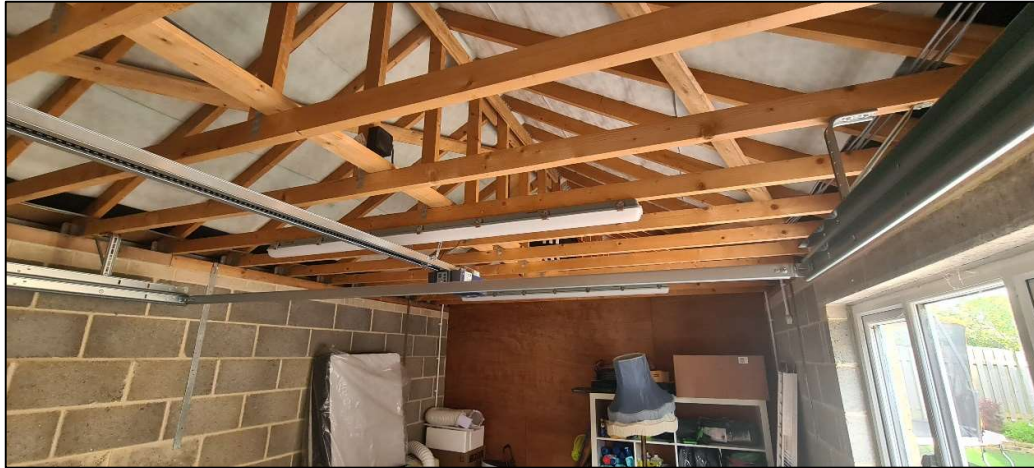
Plate 4. Internal view of the roof showing the modern prefabricated roof trusses and the breathable roofing membrane
