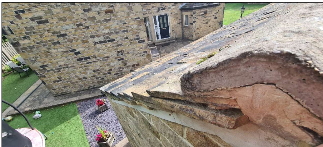
Plate 3. Gaps between the stone slates at the northern gable end.
