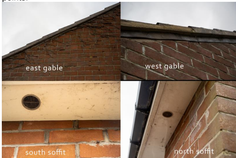
Photo 2: Gable wall and soffit details
