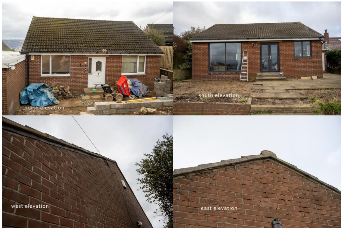
Photo 3: General view of the building
