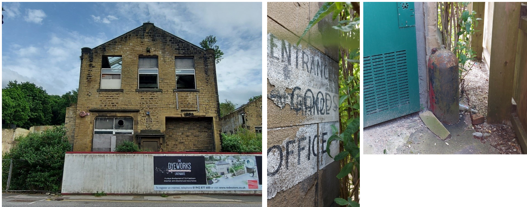
Plate 17: The front elevation, painted signage and guard stone.
