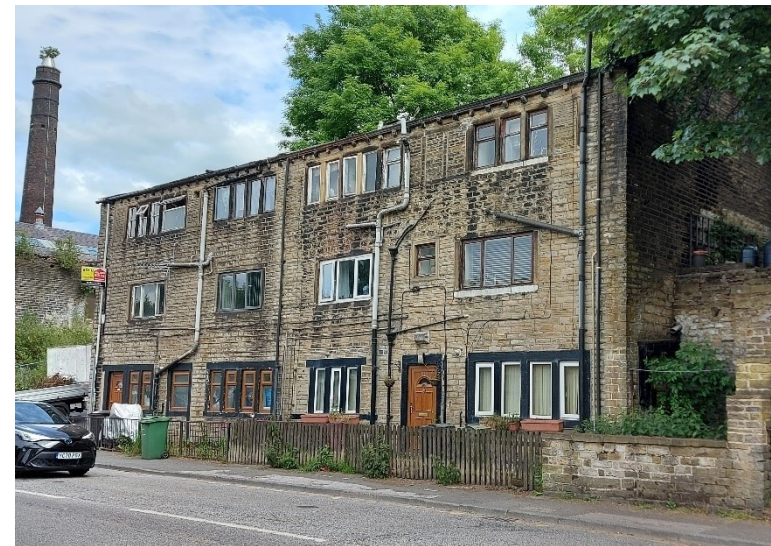
Plate 30: The mullioned windows of neighbouring cottages – with some lights infilled.
