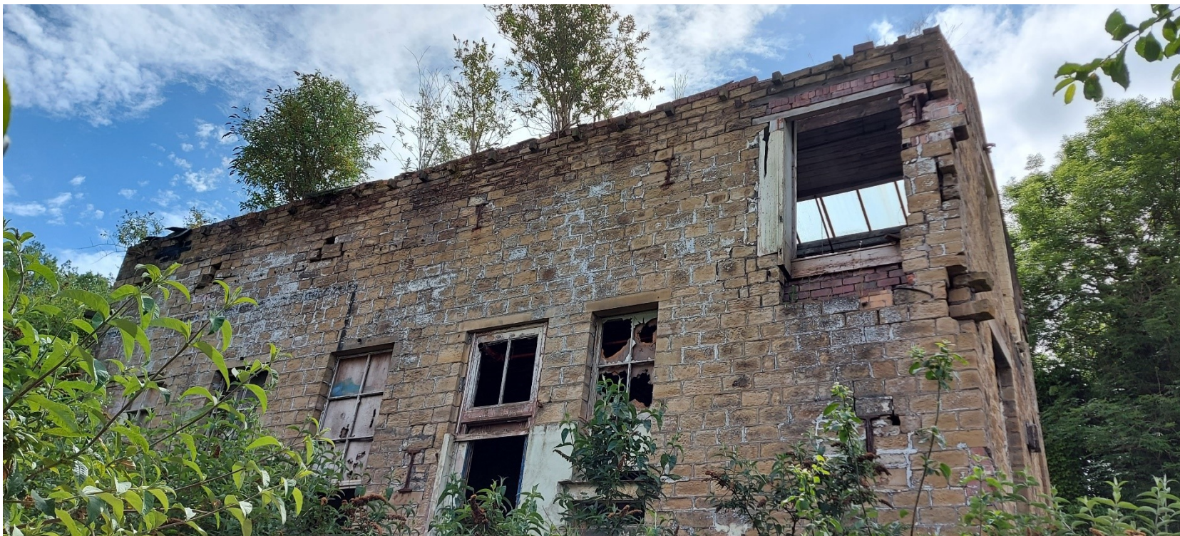
Plate 22: The northeast elevation
