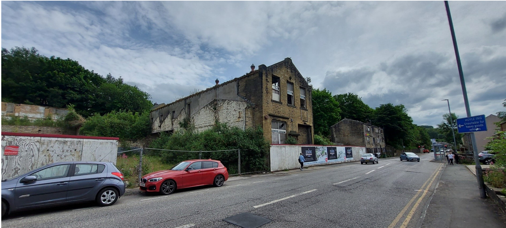
Plate 16: Building A as seen from Manchester Road.
