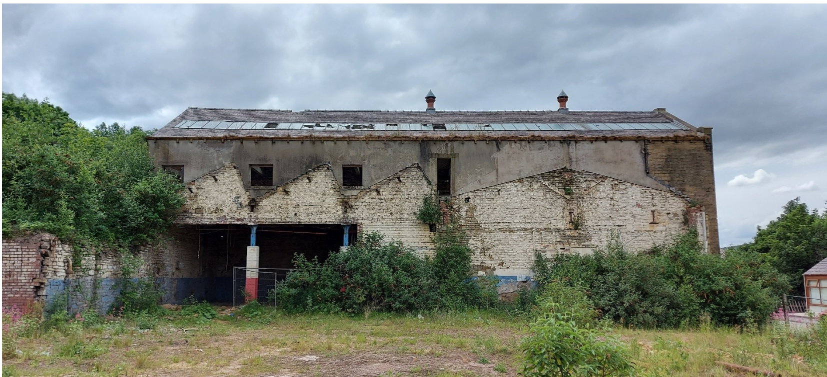
Plate 18: The northeast elevation.
