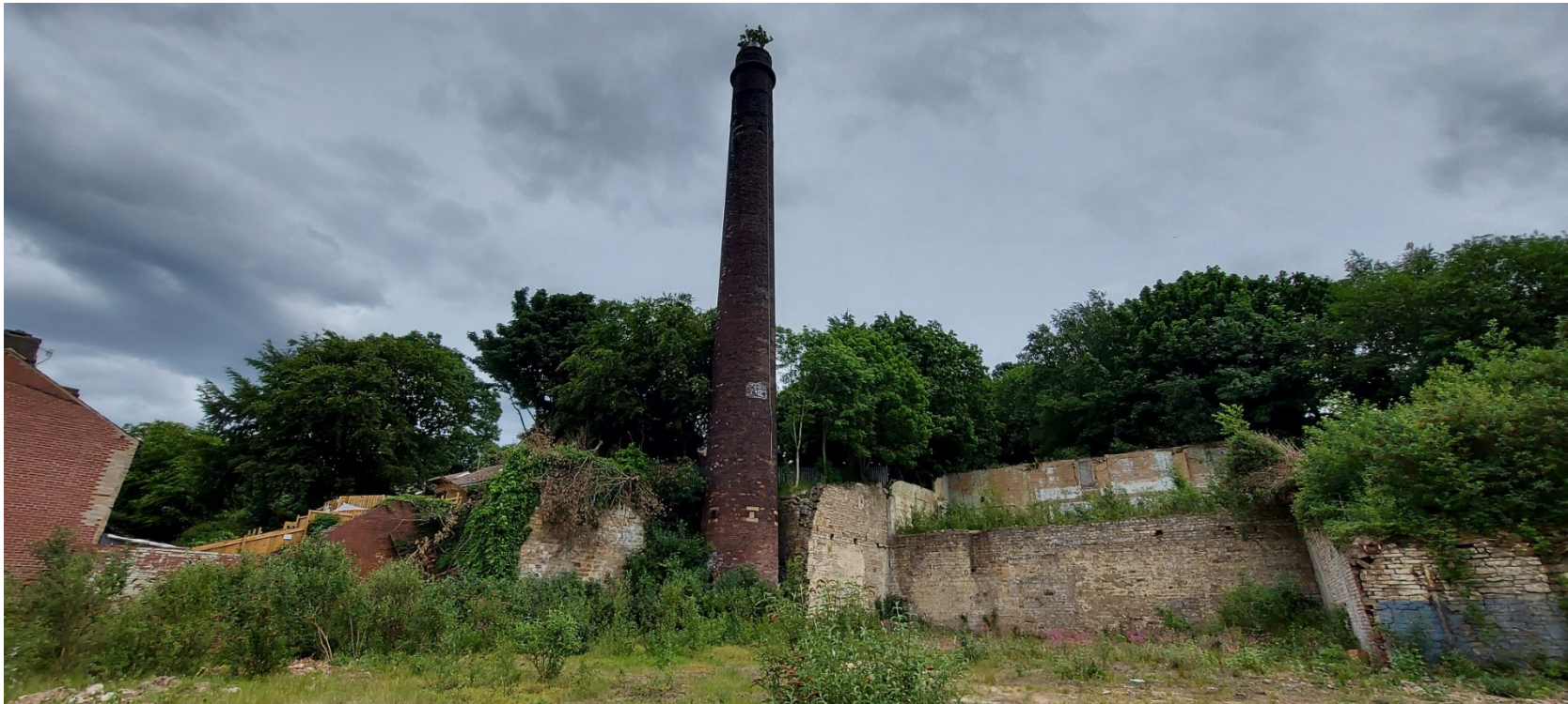
Plate 26: The circular brick chimney.
