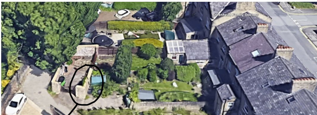
Section of wall to be removed.
