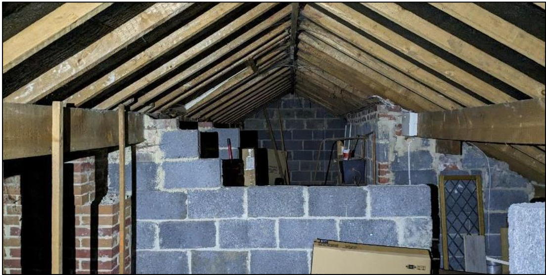
Plate 5. Roof void interior
