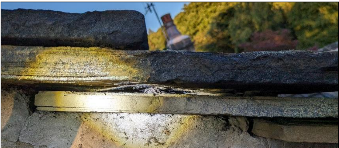
Plate 4. Example of gap between slates on verge
