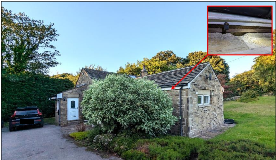
Plate 1. South corner of dwelling, with roost location behind fascia board shown in subset image
