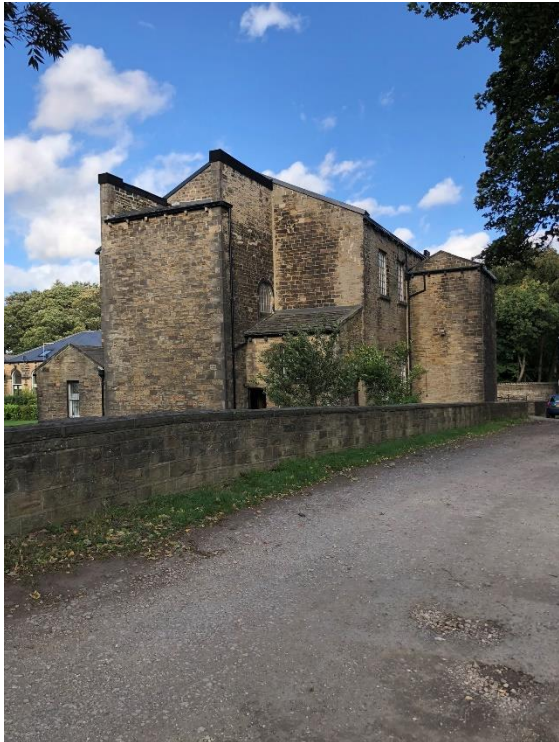
Plate 9 Rear of the Methodist chapel
