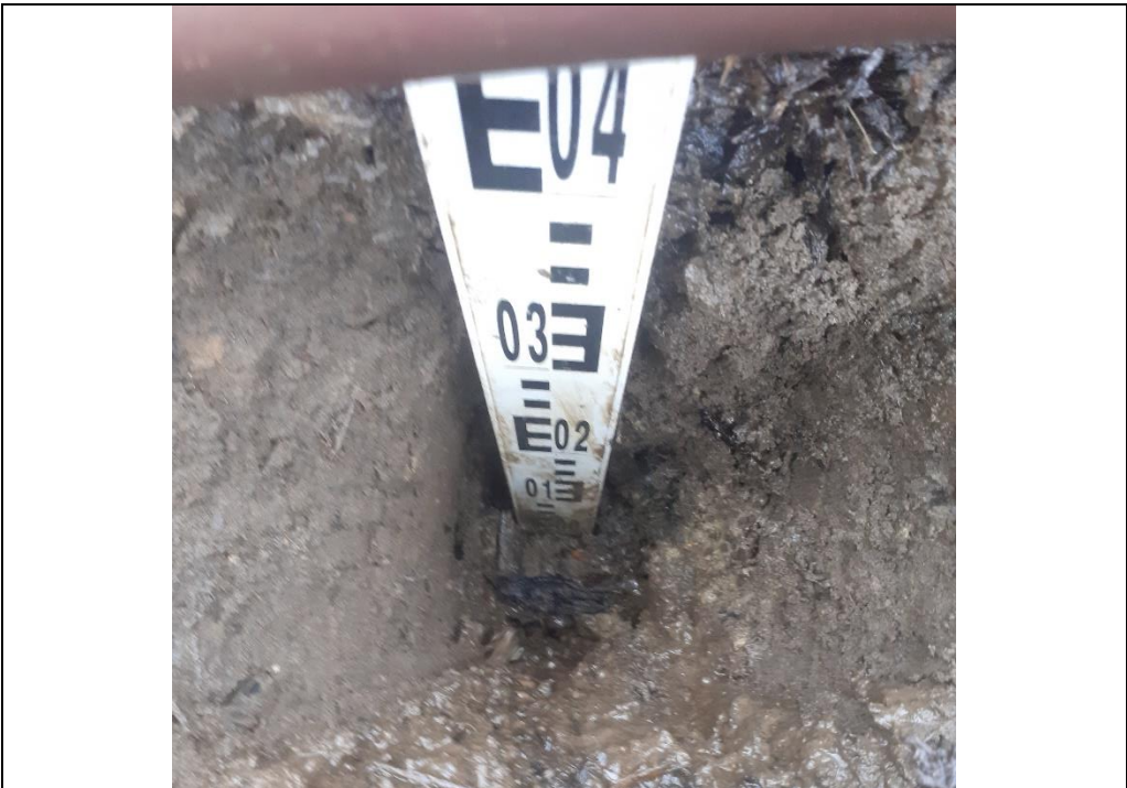
Plate 9: Photograph showing depth check in MTP303.
