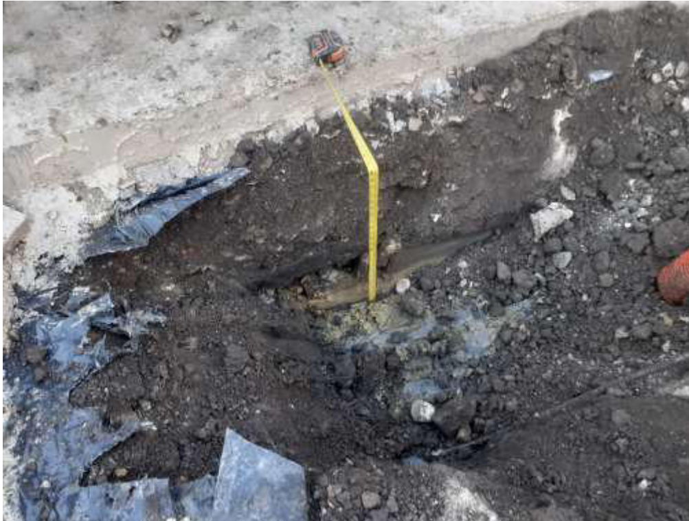
Plate 3: Picture of completed trial pit
