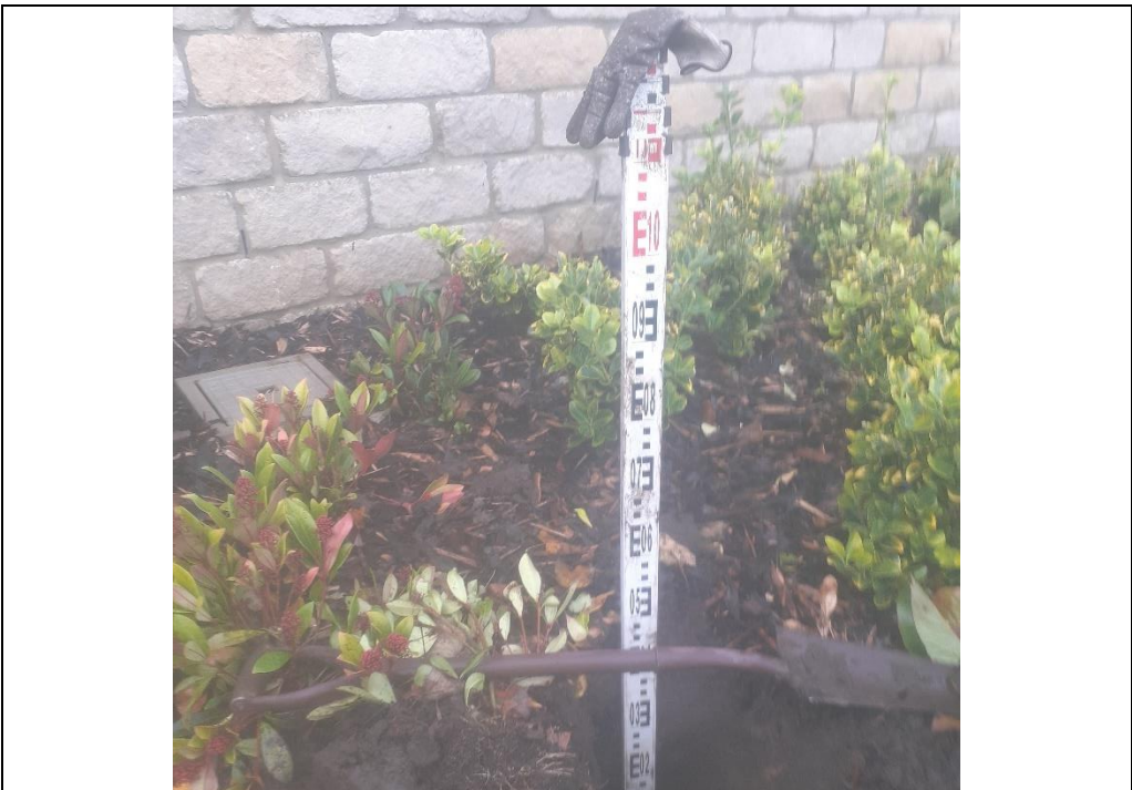
Plate 12: MTP304 Depth check showing 400 mm clean cover.
