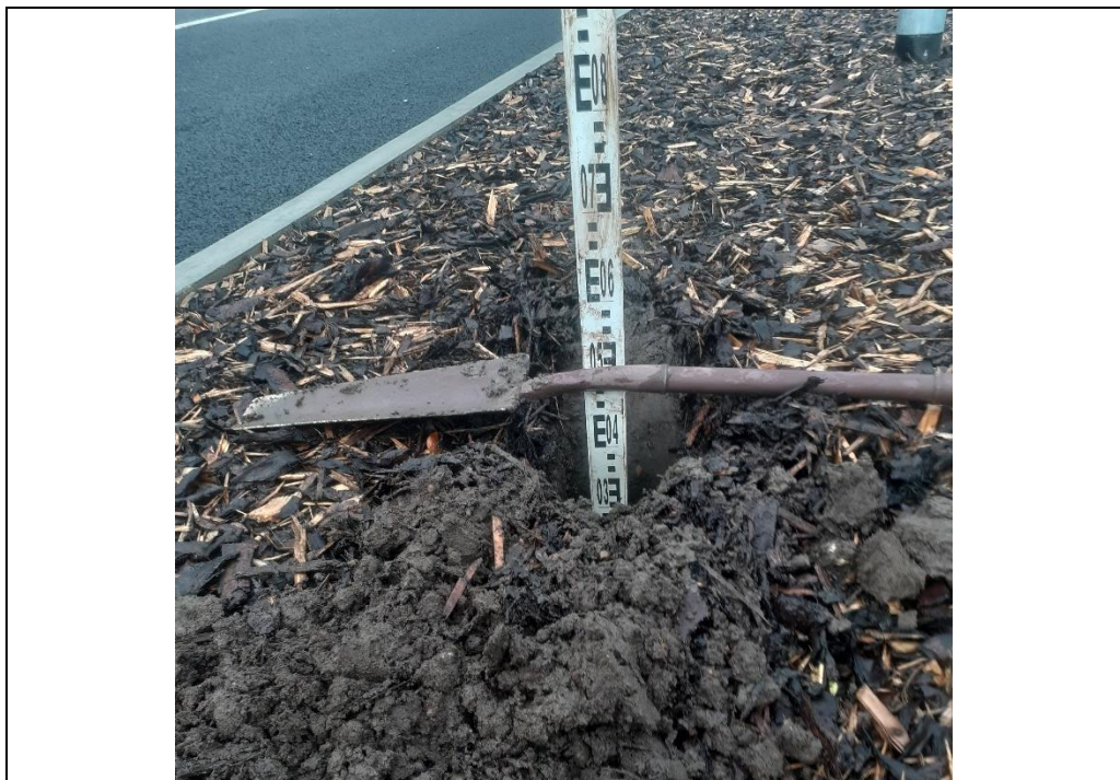
Plate 18: MTP306 Depth check showing 475 mm clean cover.
