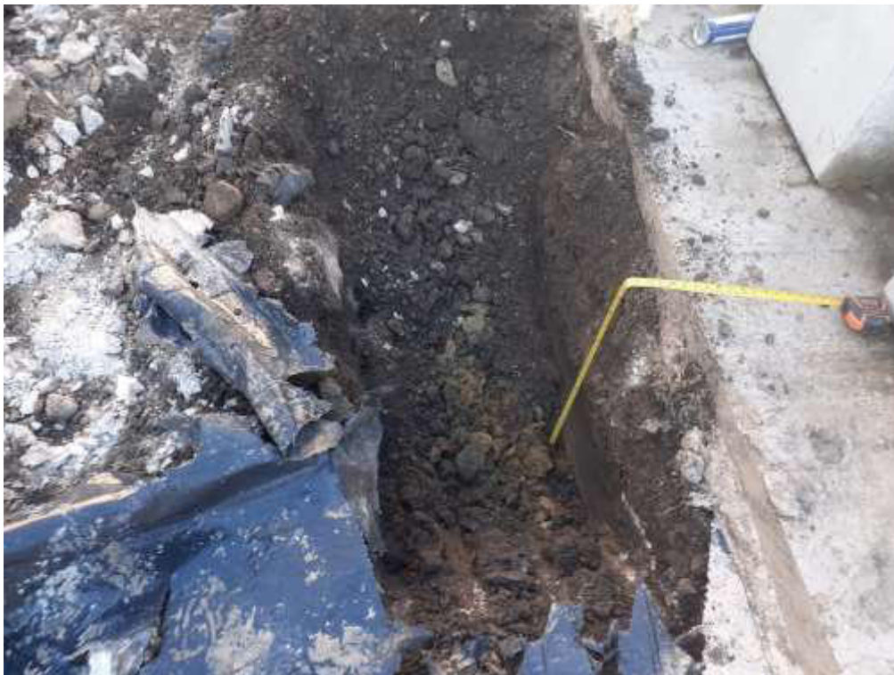
Plate 4: Picture of completed trial pit
