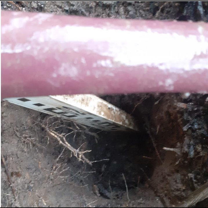
Plate 4: Photograph showing depth check in MTP301.
