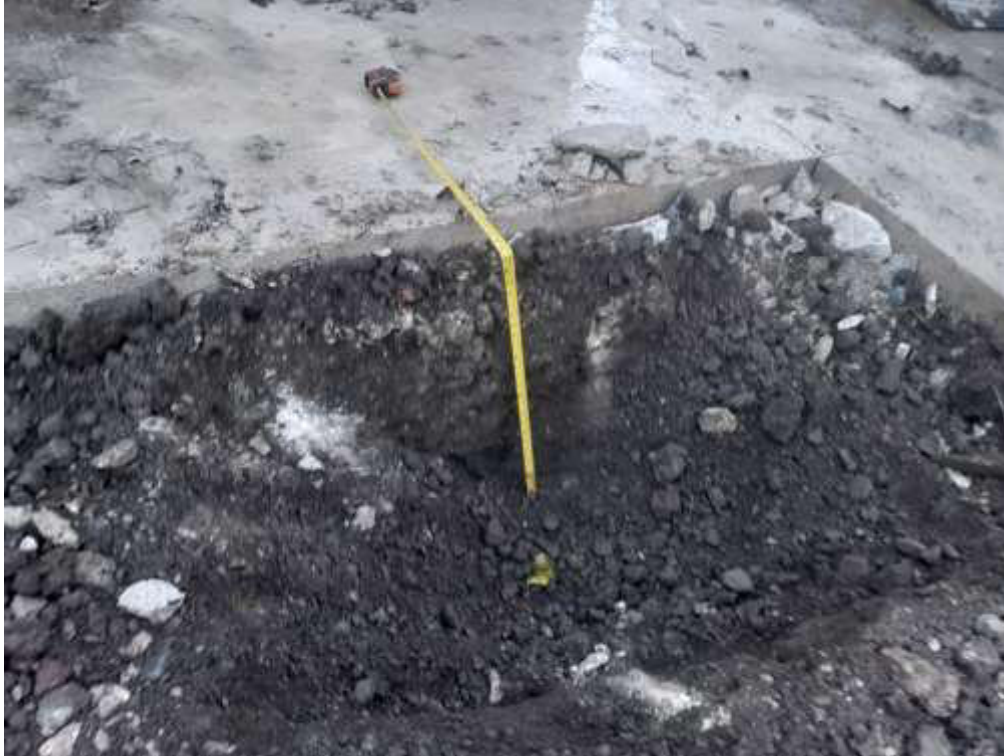
Plate 1: Picture of completed trial Pit
