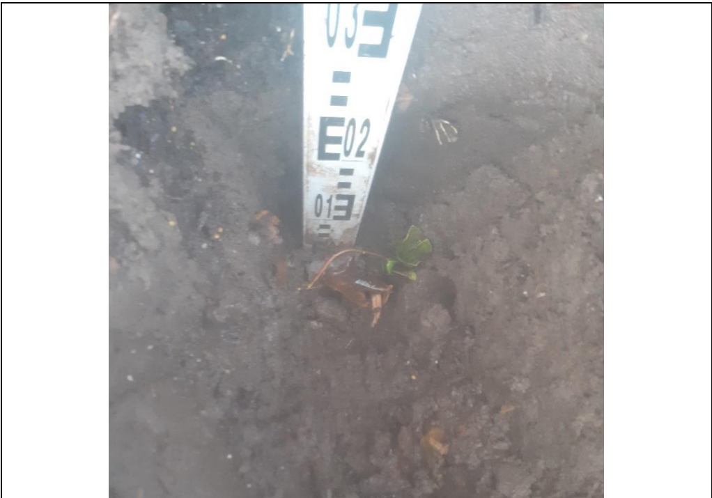
Plate 13: Photograph showing depth check in MTP304.
