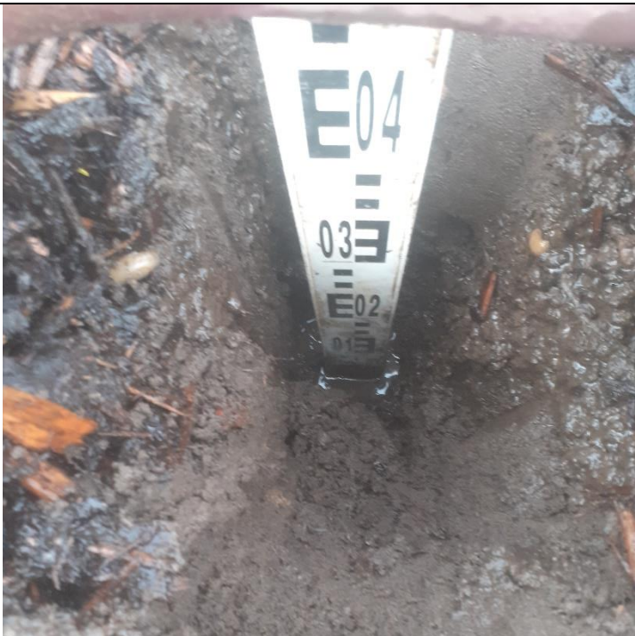
Plate 19: Photograph showing depth check in MTP306.
