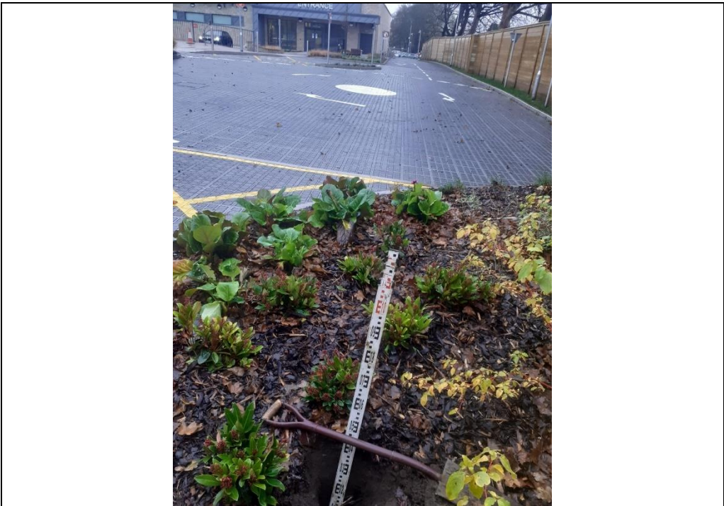
Plate 5: MTP302 verification of the depth, indicating the context of a roundabout.
