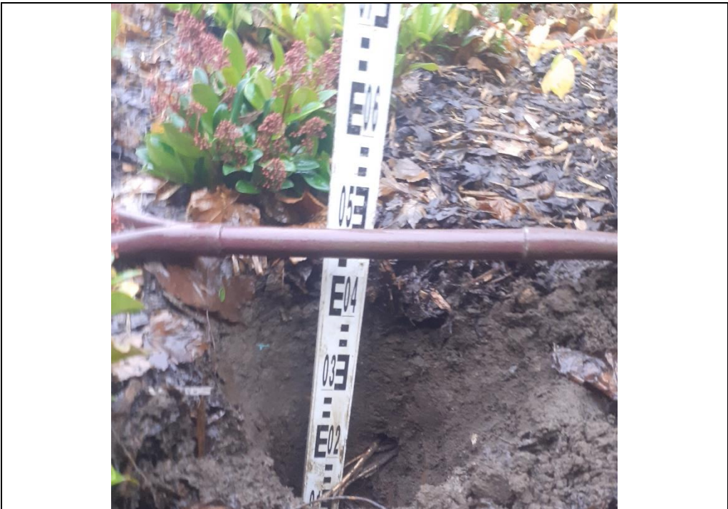
Plate 7: MTP302 Depth check showing 475 mm clean cover.
