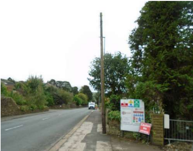
247. View of telegraph post adjacent to Wynncliff driveway. Telegraph post out of plumb/vertical alignment, leaning towards roadway by approximately 2 degrees.
