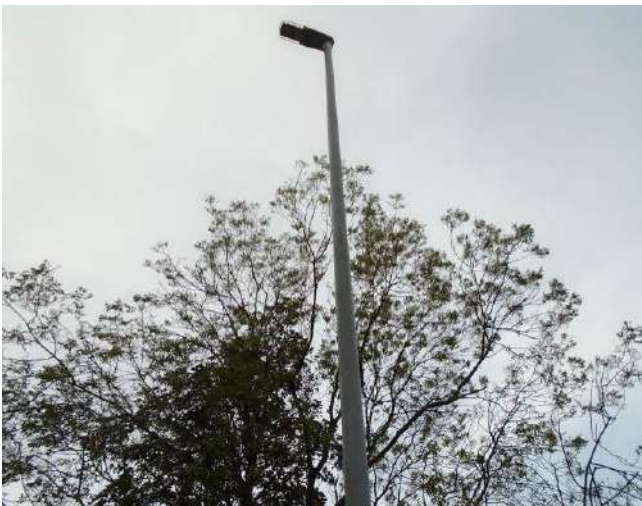
273. View of upper portion of lamp post.
