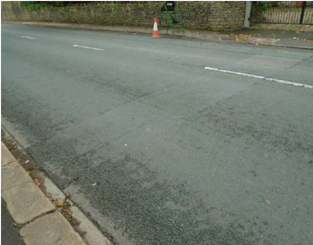
121. Patch repair to roadway.
