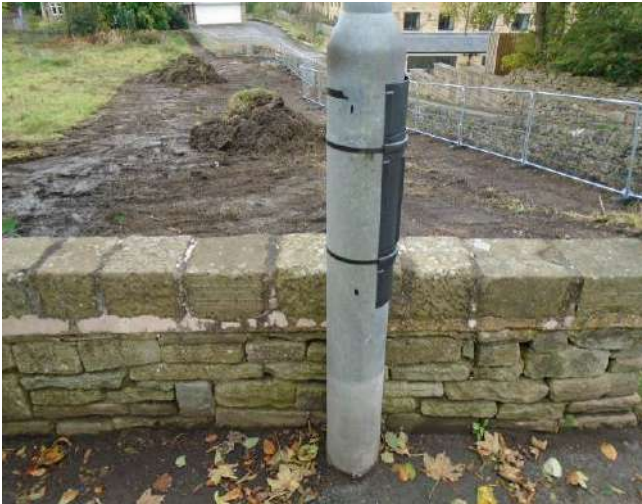
271. View of base of lamp post.
