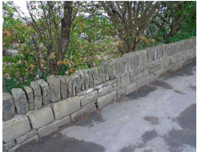
226. Dry stone wall along development site boundary.
