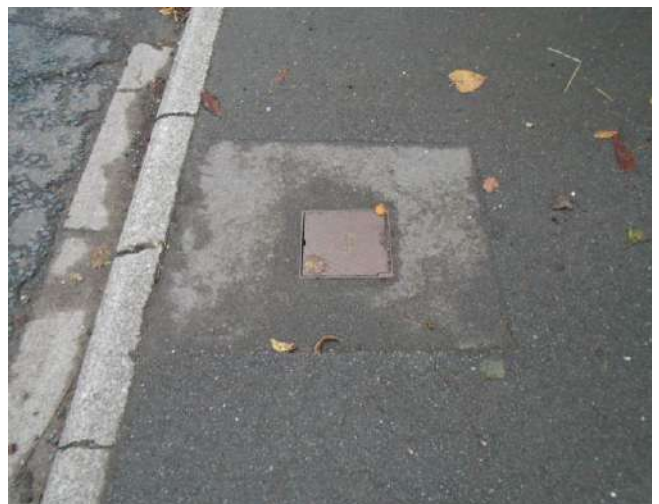
54. Patch repair to water main location.
