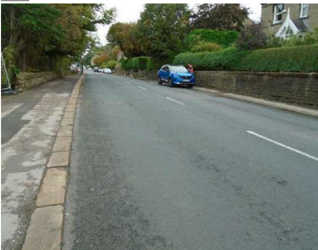
107. General view along carriageway.
