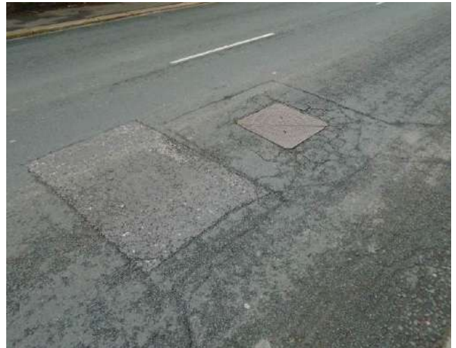
88. Patch repair to tarmacadam.
