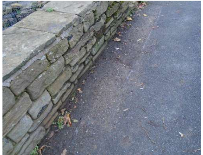
206. Worn tarmac surfacing adjacent to inspection chamber.
