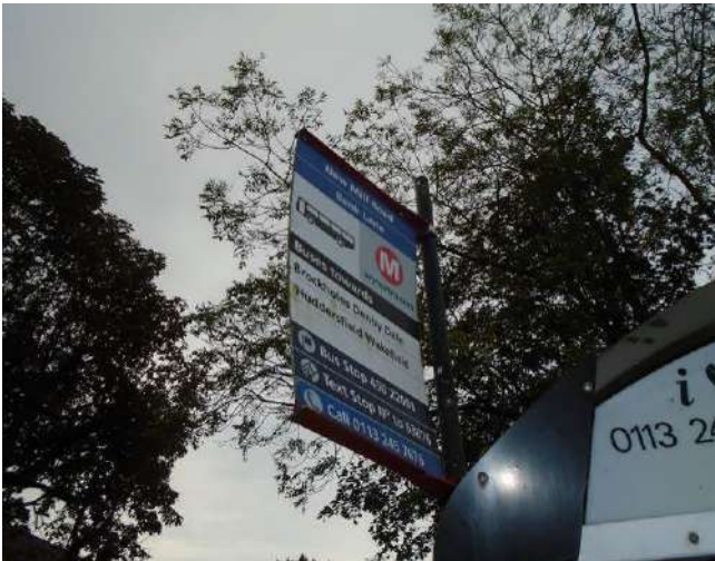
267. Impact damage and disturbed decorations to bus shelter sign and associated post.
