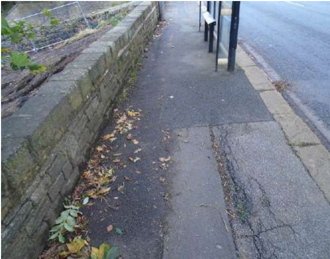
193. Assorted ages of tarmacadam present to footpath surface.
