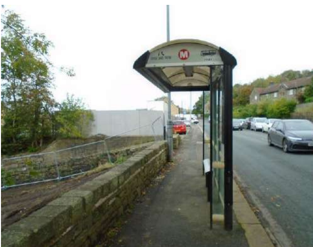
257. View of southern elevation of bus shelter.
