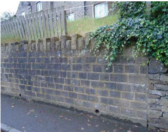
39. Coursed stone boundary wall to elevated properties.
