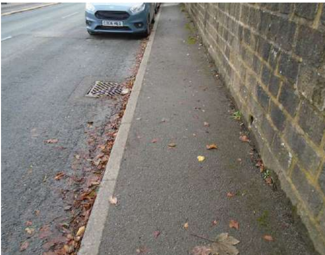
77. View of tarmac to pavement.
