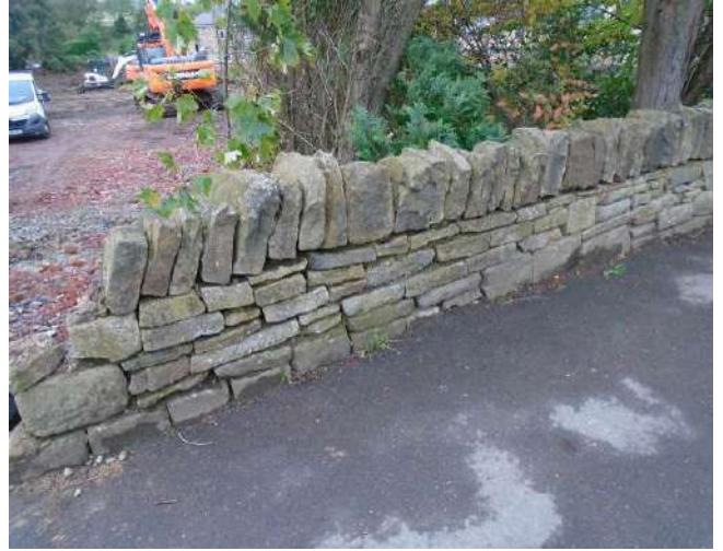
224. View of dry stone wall at boundary to development site.
