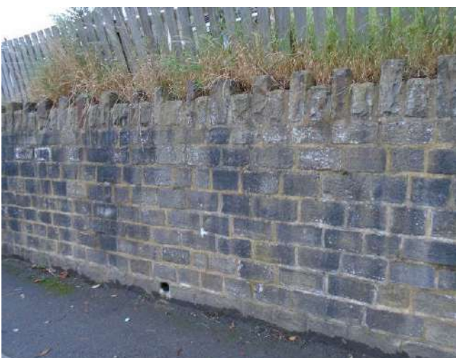
41. Coursed stone boundary wall to elevated properties.
