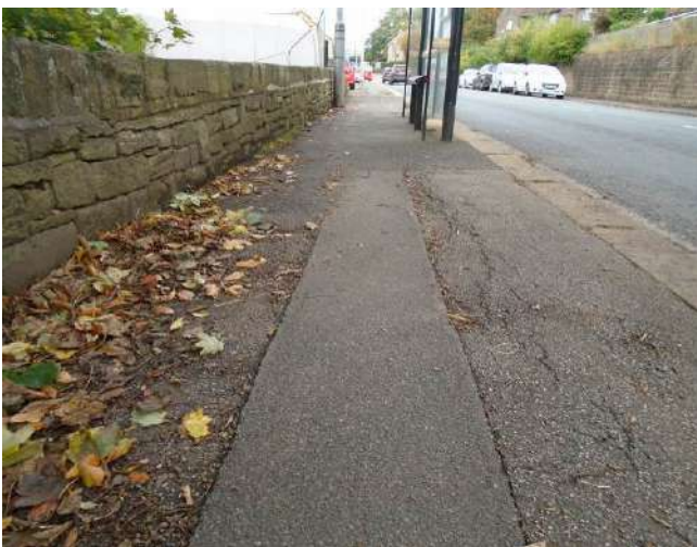
191. Scars and splits/cracks to tarmacadam surface. Paving is uneven approaching bus shelter.
