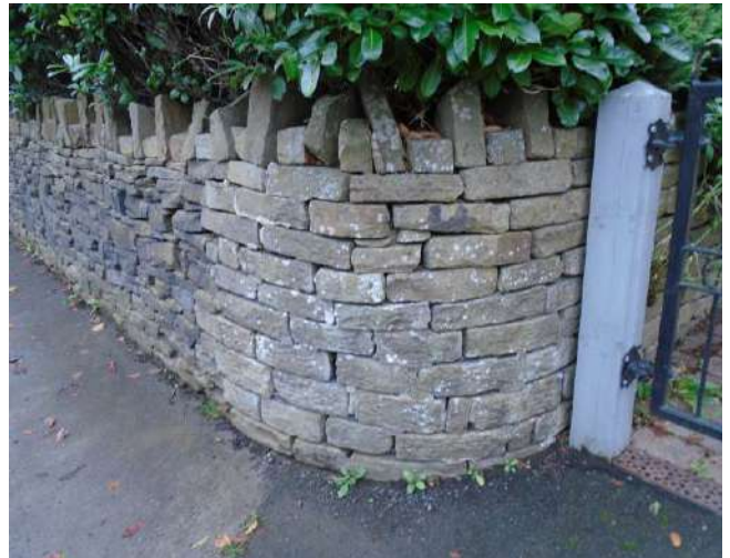
28. View of return wall to 6A.
