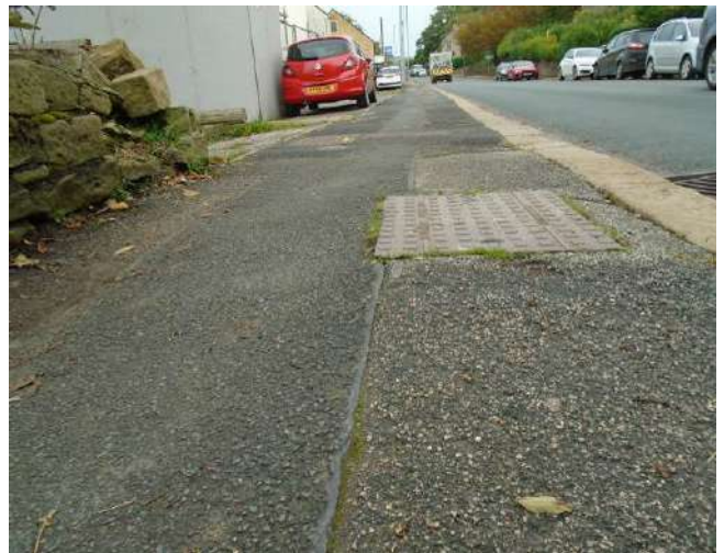
208. View across inspection chamber.
