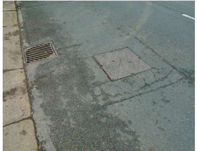
110. Patch repairs around chamber in gateway to development site.
