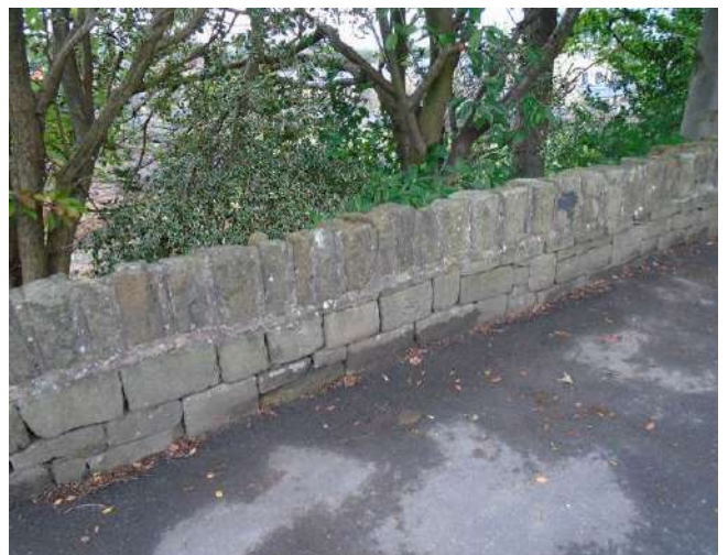
228. Boundary wall to development site.
