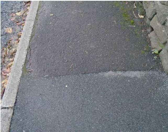
57. View of joint between resurfaced area and original footpath.
