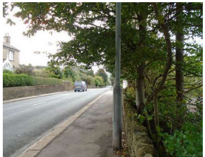
252. View of base of lamp post. Lamp post is slightly out of plumb, leaning inwards towards the development site by approximately 2 degrees.
