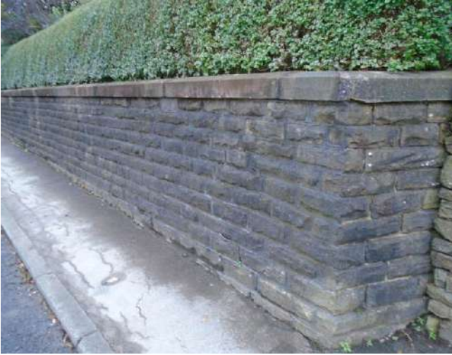
1. View of boundary wall.
