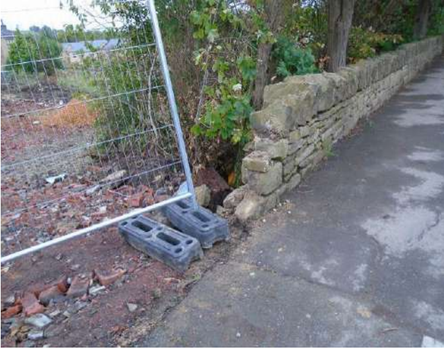
223. Section of boundary wall taken down to development site entrance.
