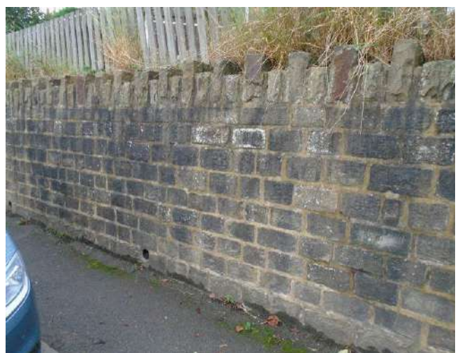
42. Coursed stone boundary wall to elevated properties.
