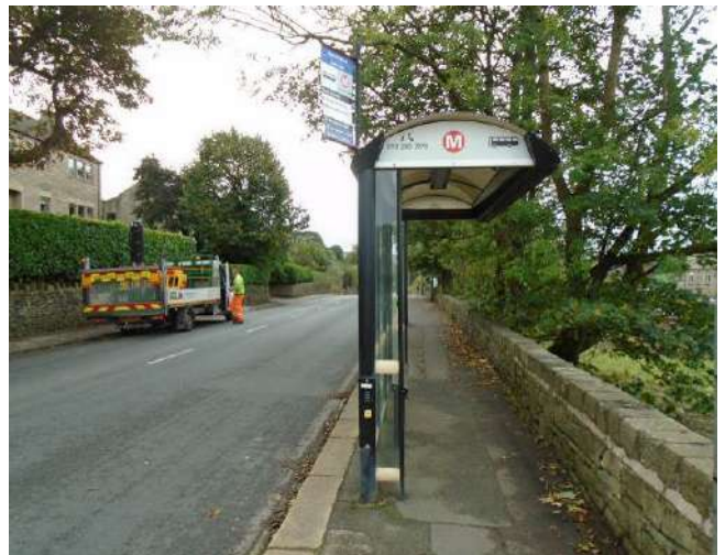
262. View of northern elevation of bus shelter.
