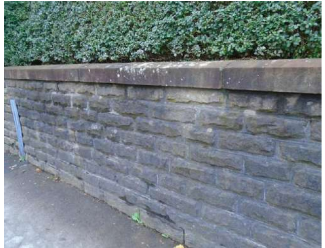
8. View of boundary wall.
