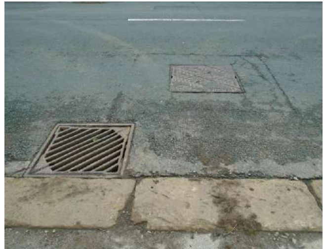
112. View of gully and chamber in entrance to development site.
