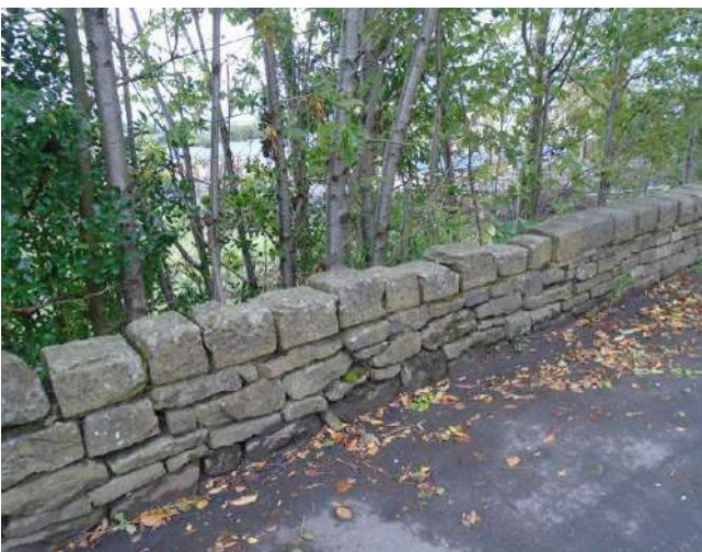
233. Dry stone boundary wall to development site.
