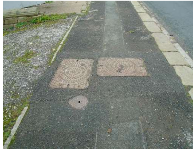
212. Views of inspection chambers.
