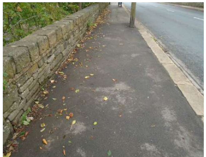
180. View of tarmacadam footpath.
