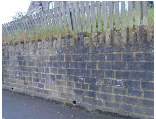
40. Coursed stone boundary wall to elevated properties.
