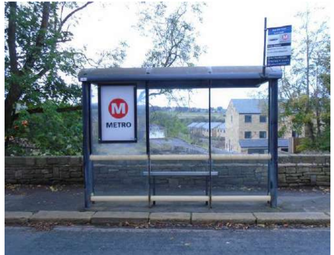
268. View of eastern elevation of bus shelter.
