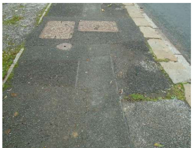
210. Uneven, disturbed and worn tarmac surfacing including patch repairs within entrance area into property adjoining development site, 'Glen View'.
