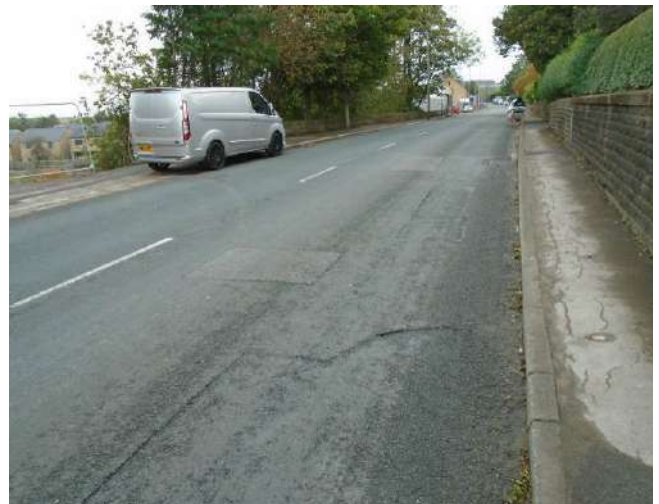
78. General view along carriageway.
