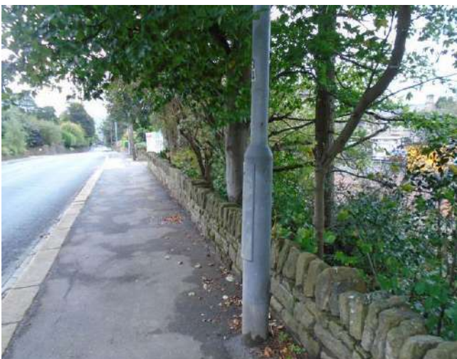
251. View of base of lamp post. Lamp post is slightly out of plumb, leaning inwards towards the development site by approximately 2 degrees.
