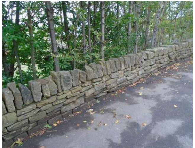
232. Dry stone boundary wall to development site.
