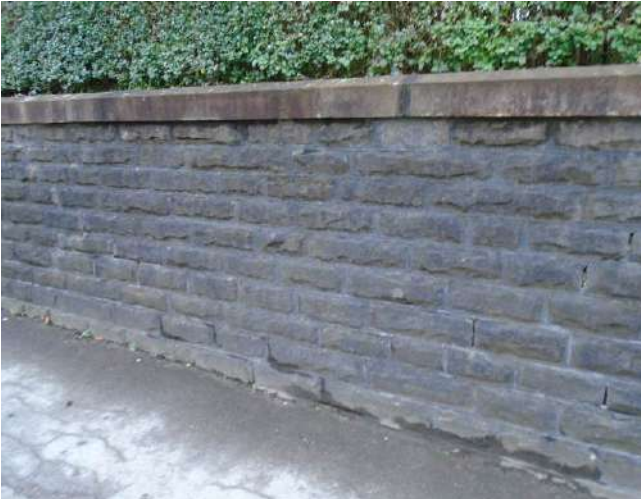
3. View of boundary wall.
