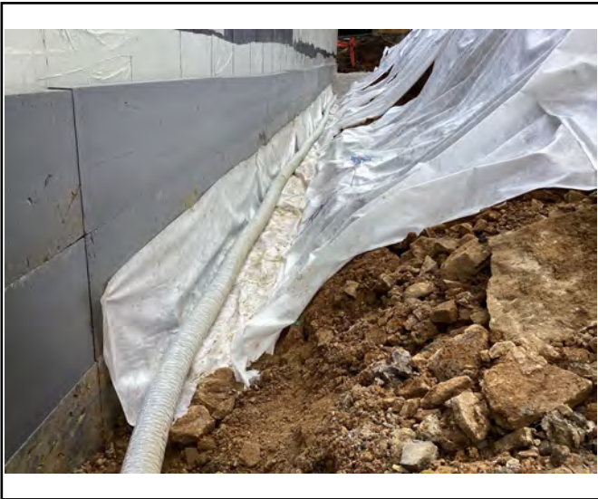
View of a land drain at the base of the retaining wall.
