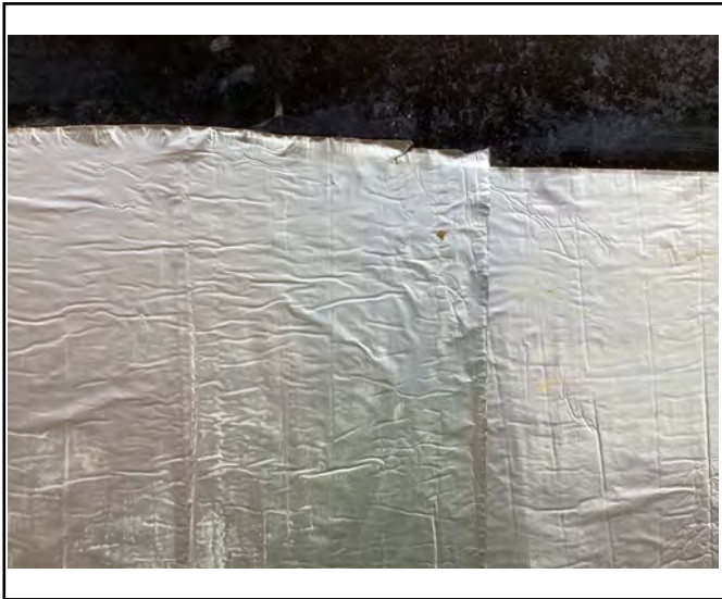
View showing both the bitumen primer and applied GRSAM
