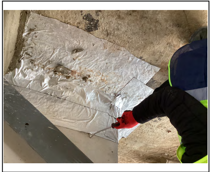
View of a concrete base requiring priming prior to sealing with GRSAM
