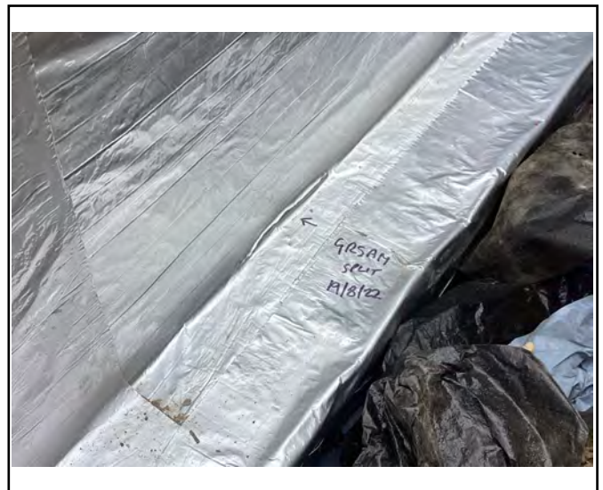
Butyl Tape being installed during
