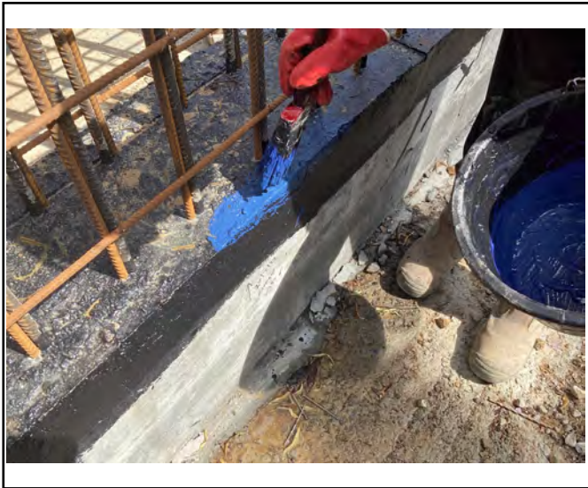
Application of Liquid Gas Membrane
