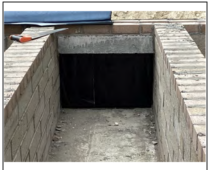
View of one of two sections of wall which will be completed later.
