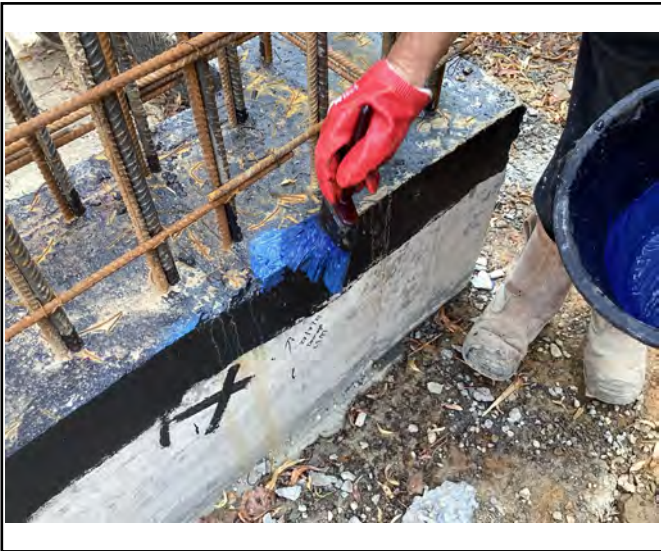
Application of Liquid Gas Membrane
