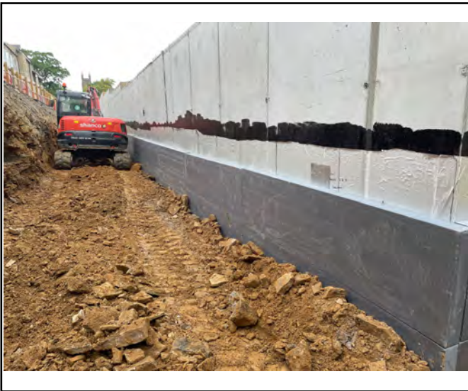
Alternative view of insulation protecting GRSAM along rear of retaining wall
