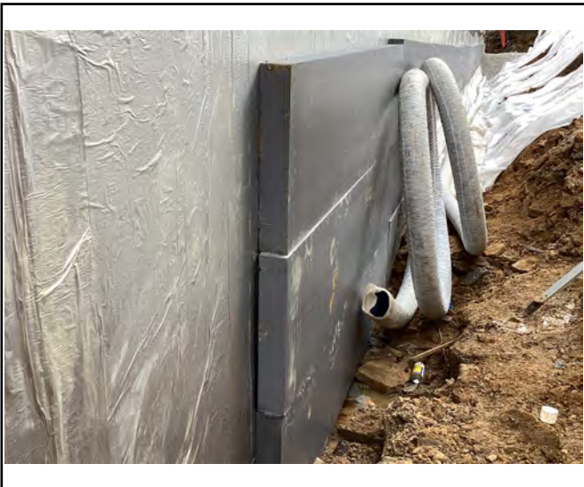
View showing both the land drain and insulation protecting the GRSAM
