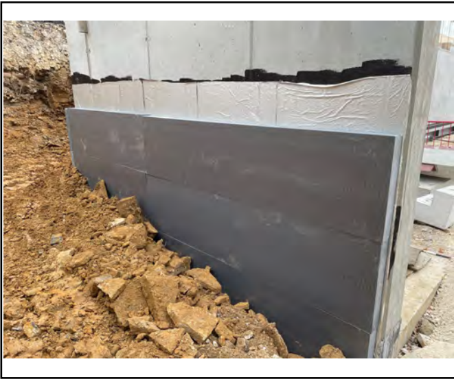
View of insulation protecting the GRSAM along rear of retaining wall
