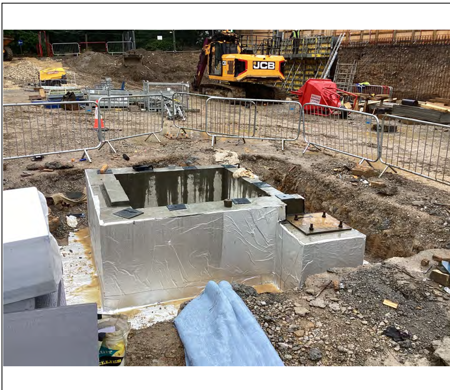
Alternative overview of the Lift Pit - the verified area
