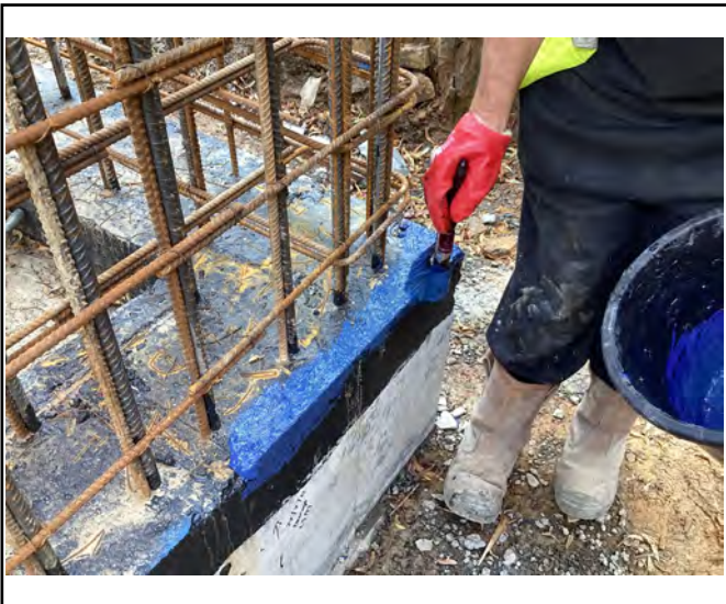
Application of Liquid Gas Membrane
