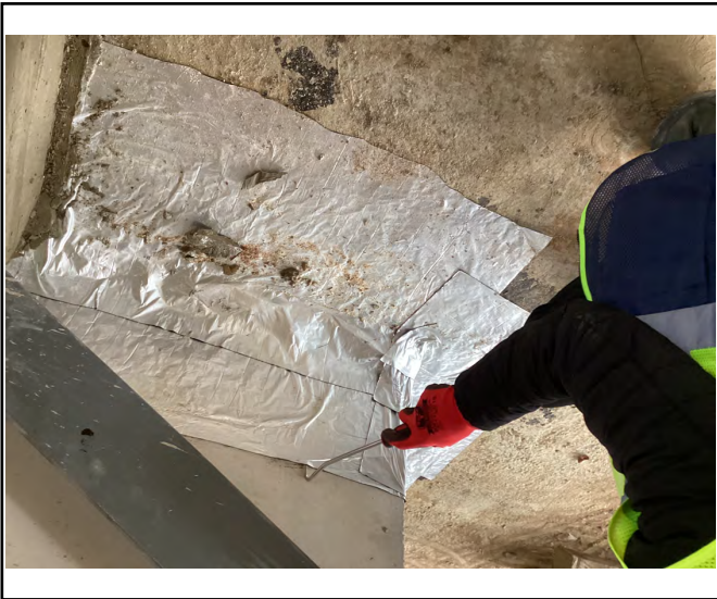
View showing where the concrete slab thickens.
