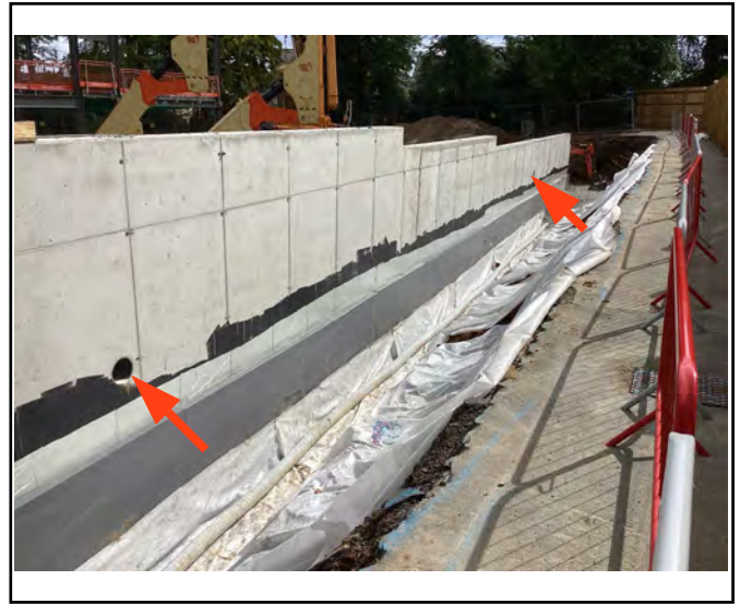
View showing the positions of the ducts requiring sealing
