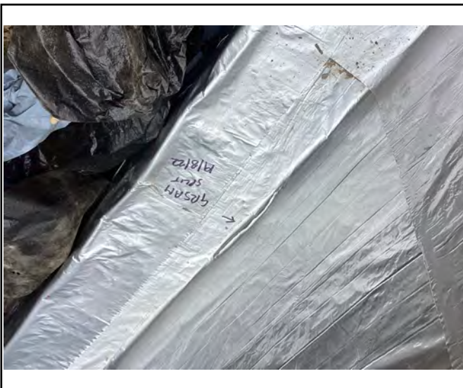
Detailing to toe using GRSAM being
