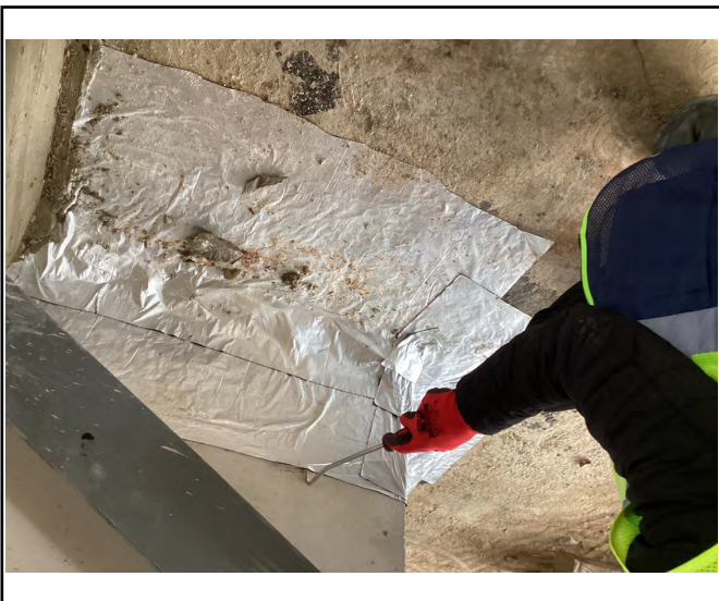
View of incomplete substrate
