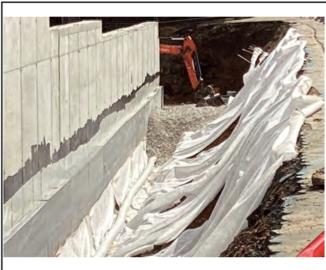
View of backfill against the insulation
