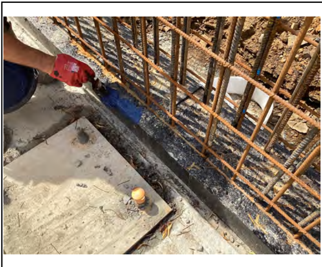
Application of Liquid Gas Membrane
