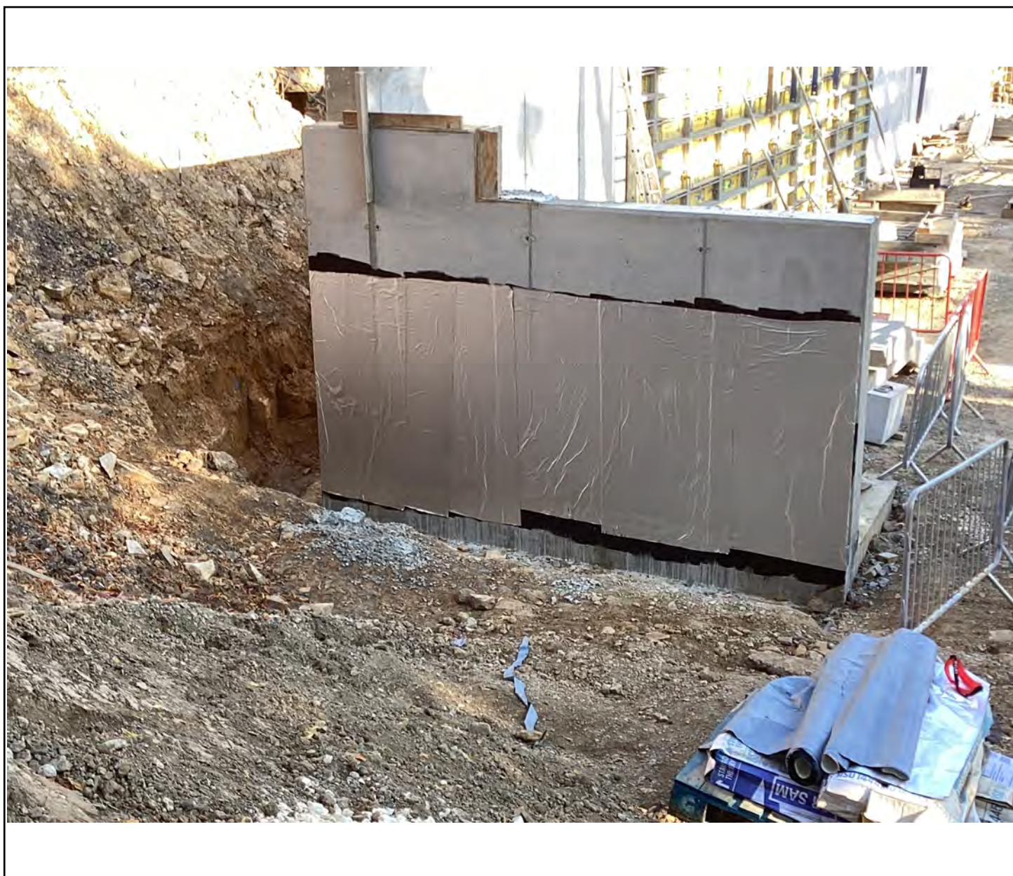
Alternative overview of the Retaining Wall return
