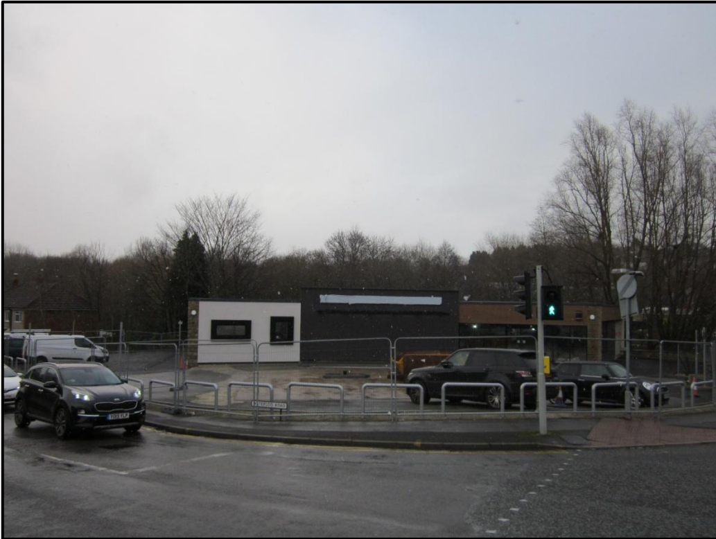
Photograph 1. Location of the new food takeaway business
