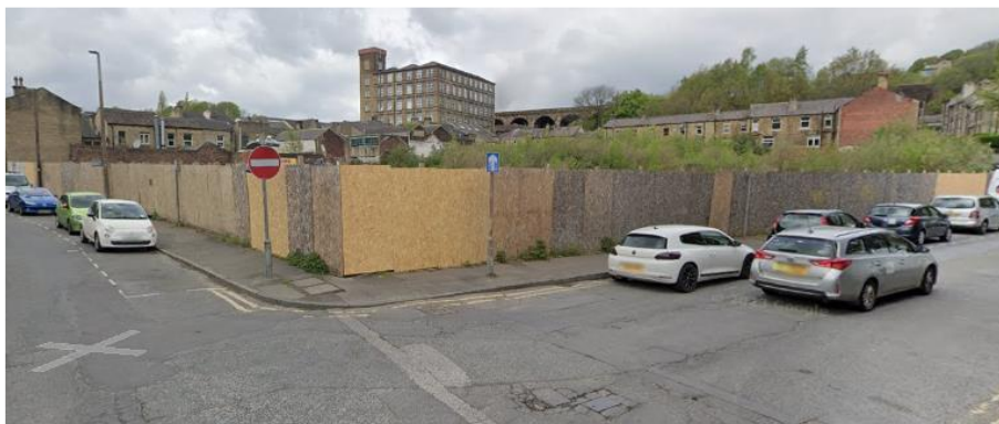
Figure 1 Street view of site
