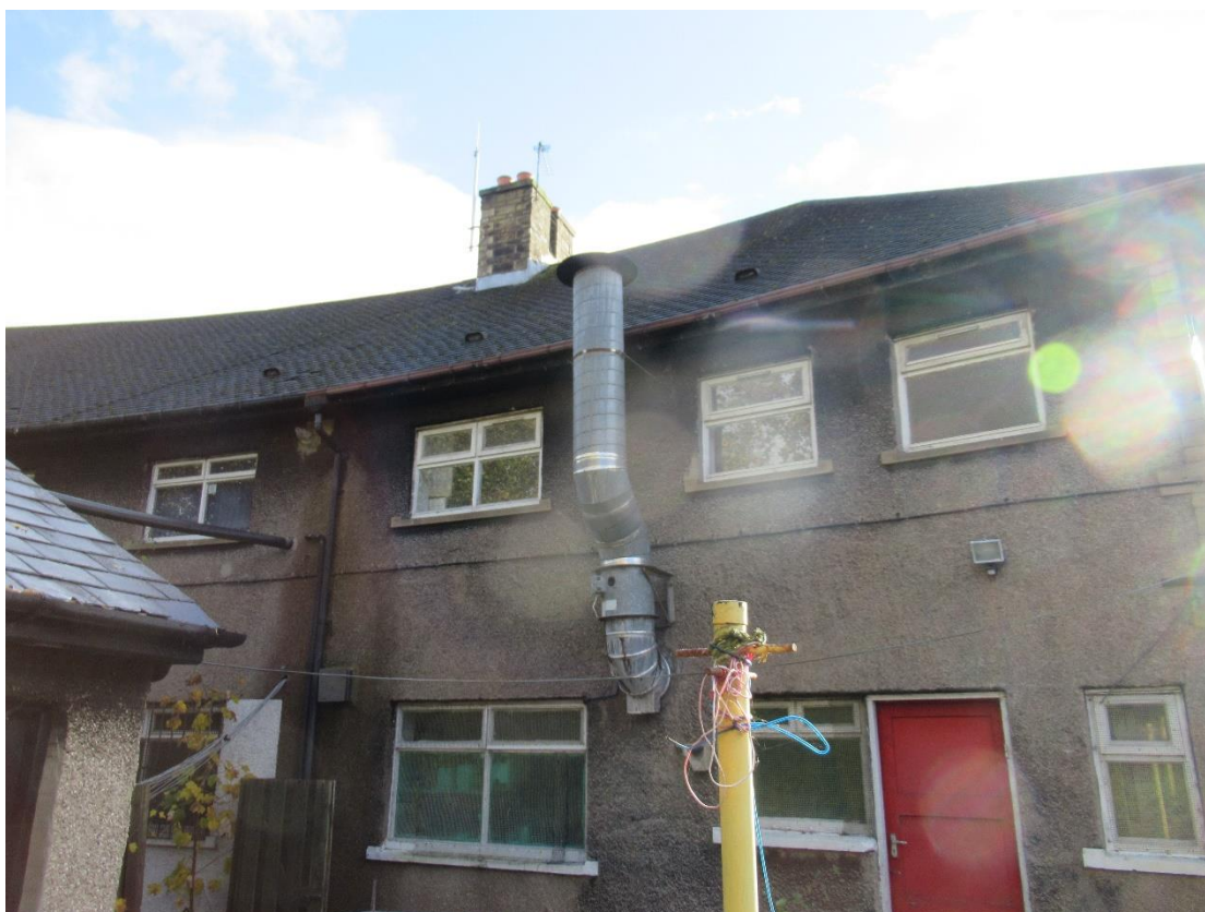
Photograph 5 - External view of westernmost end of northwestern aspect of Building 1.
