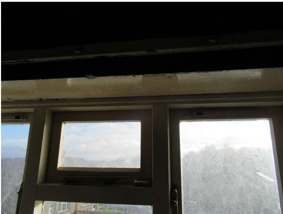
Photograph 12 – Internal view of window in Building 1.
