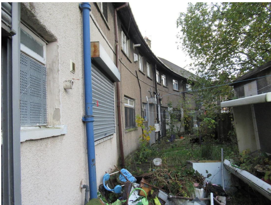
Photograph 3 - External view of northwestern aspect of Building 1.
