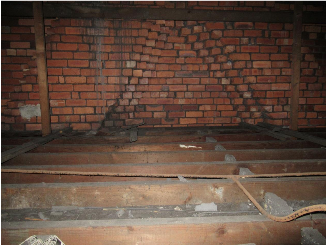
Photograph 23 – Loft Space 4 in Building 1.
