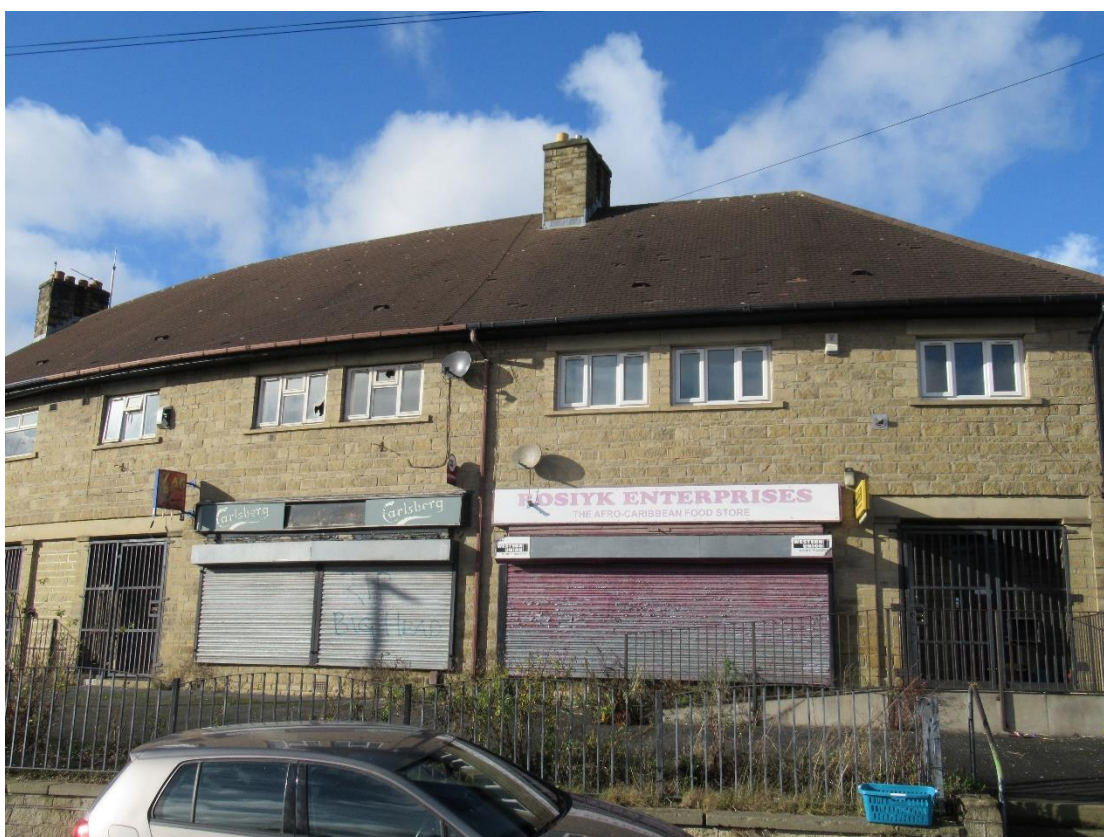
Photograph 2 - External view of southeastern aspect of Building 1.
