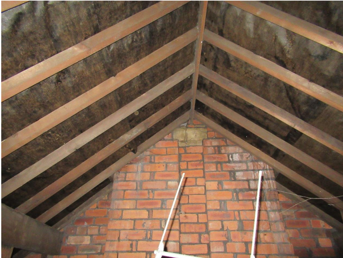
Photograph 13 – Gable end of Loft Space 1 in Building 1.
