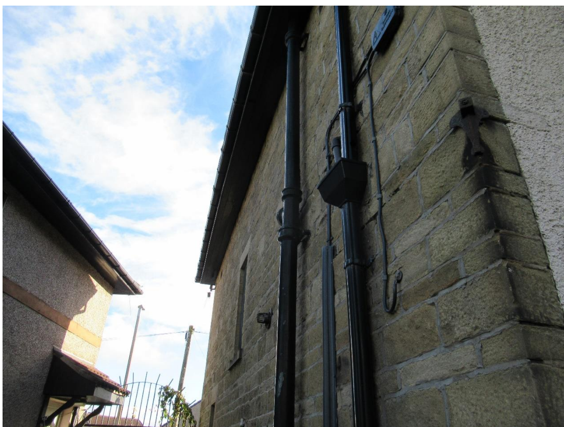
Photograph 6 - External view of northeastern aspect of Building 1.
