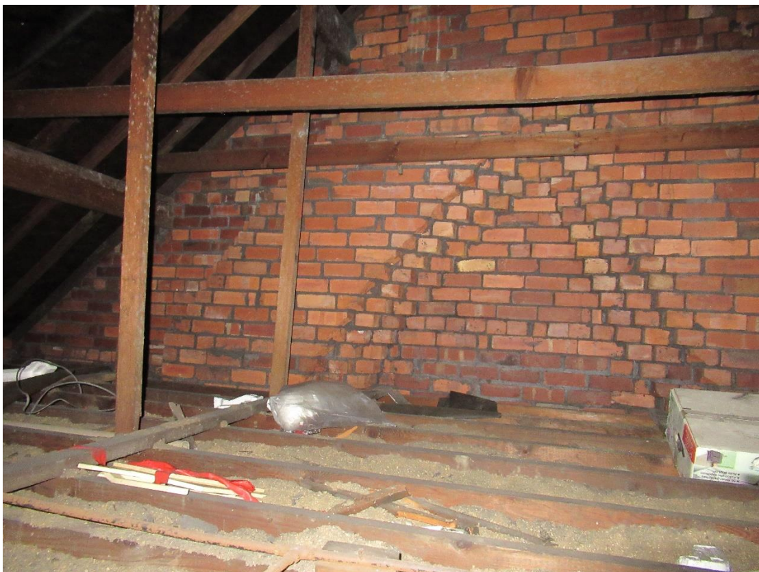
Photograph 20 – Loft Space 3 in Building 1.
