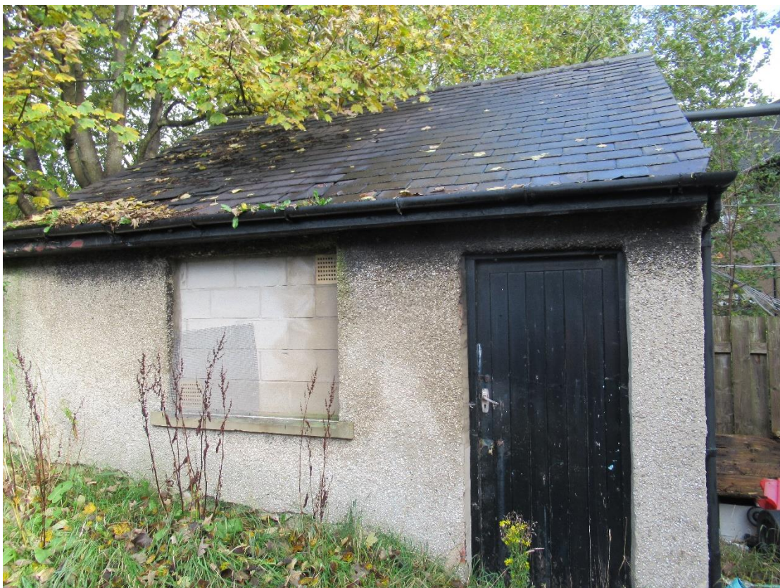
Photograph 30 - External view of southwest aspect of Building 3.
