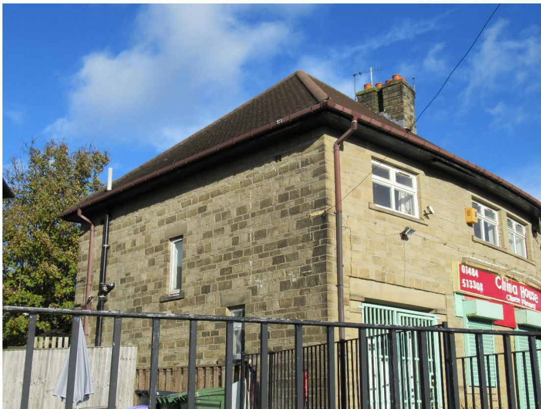
Photograph 1 – External view of southwestern aspect of Building 1.
