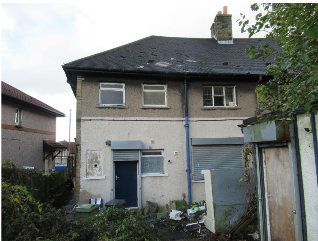
Photograph 4 - External view of easternmost end of northwestern aspect of Building 1.
