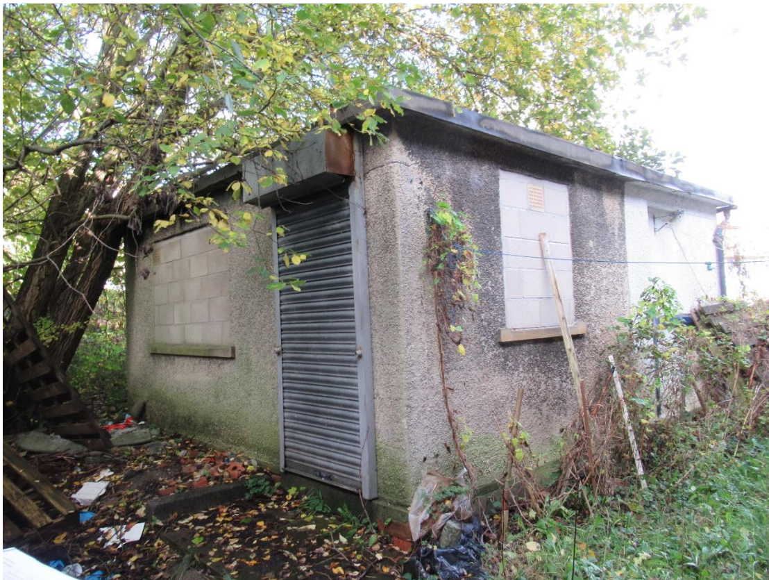
Photograph 26 – External view of southwestern aspect of Building 2.
