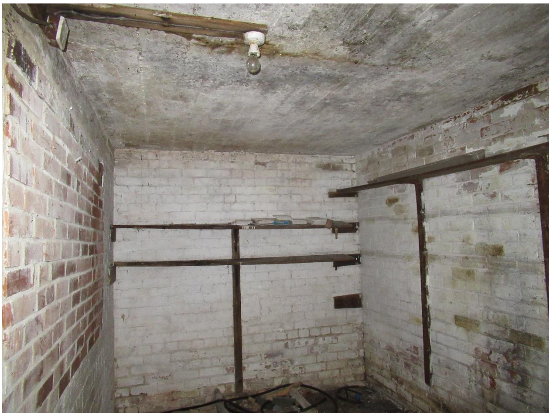
Photograph 28 – Internal view of Building 2.
