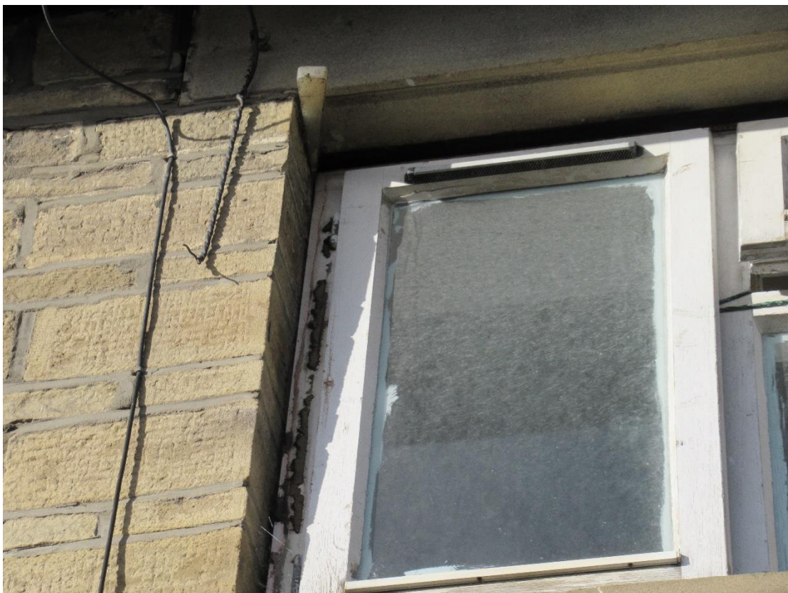
Photograph 10 – External view of window on Building 1.
