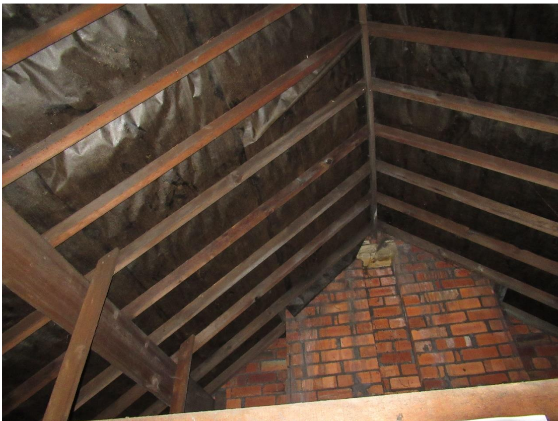
Photograph 18 – Bitumen felt in roof of Loft Space 2 in Building 1.
