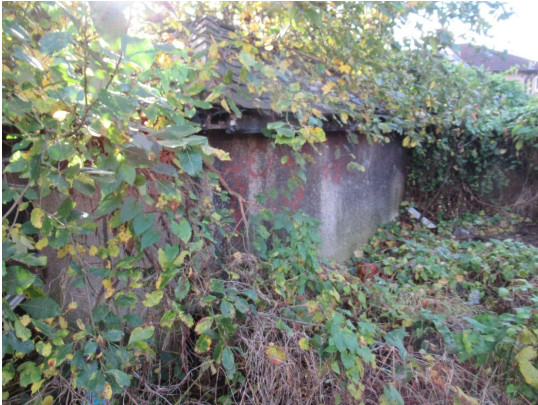
Photograph 31 - External view of northwestern aspect of Building 3.
