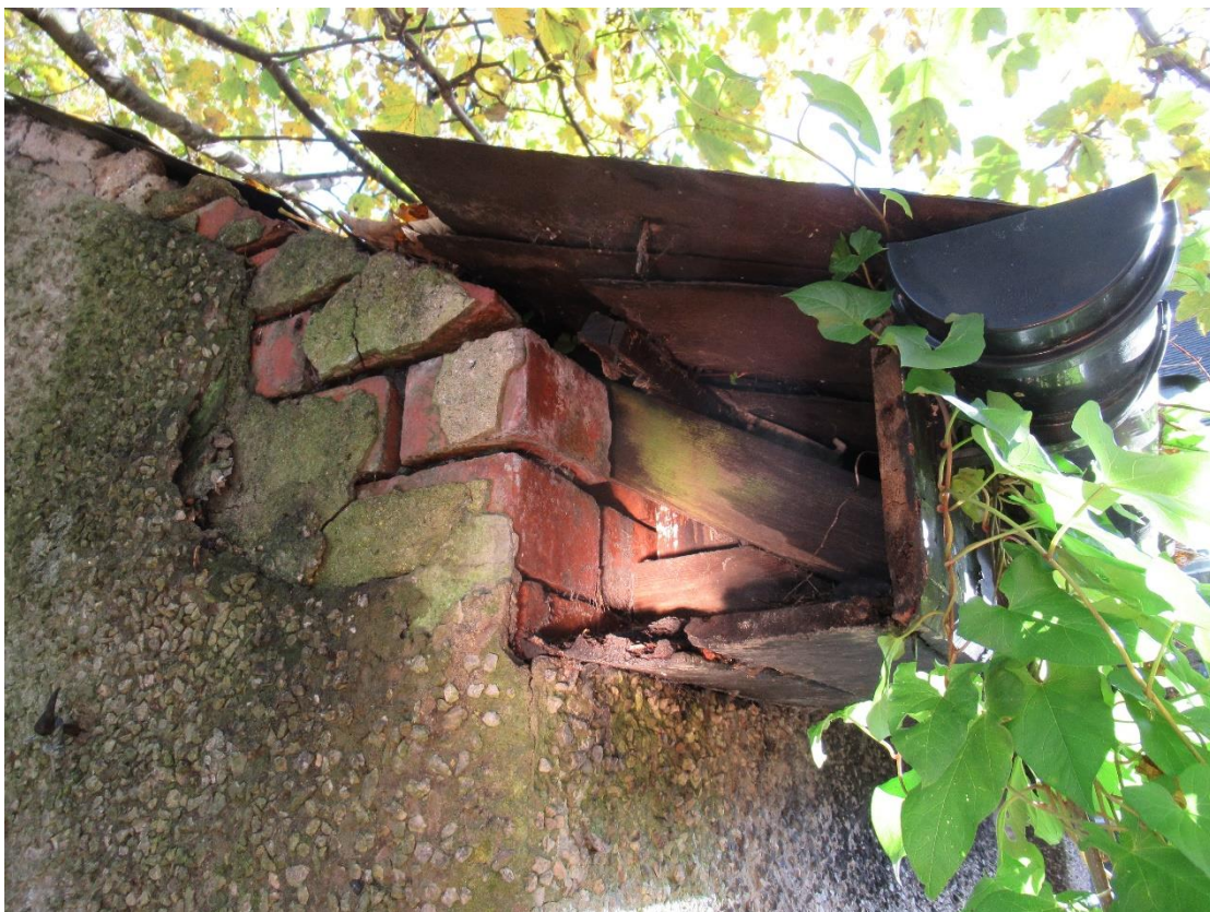
Photograph 36 – Opening into soffit box at gable end of Building 3.
