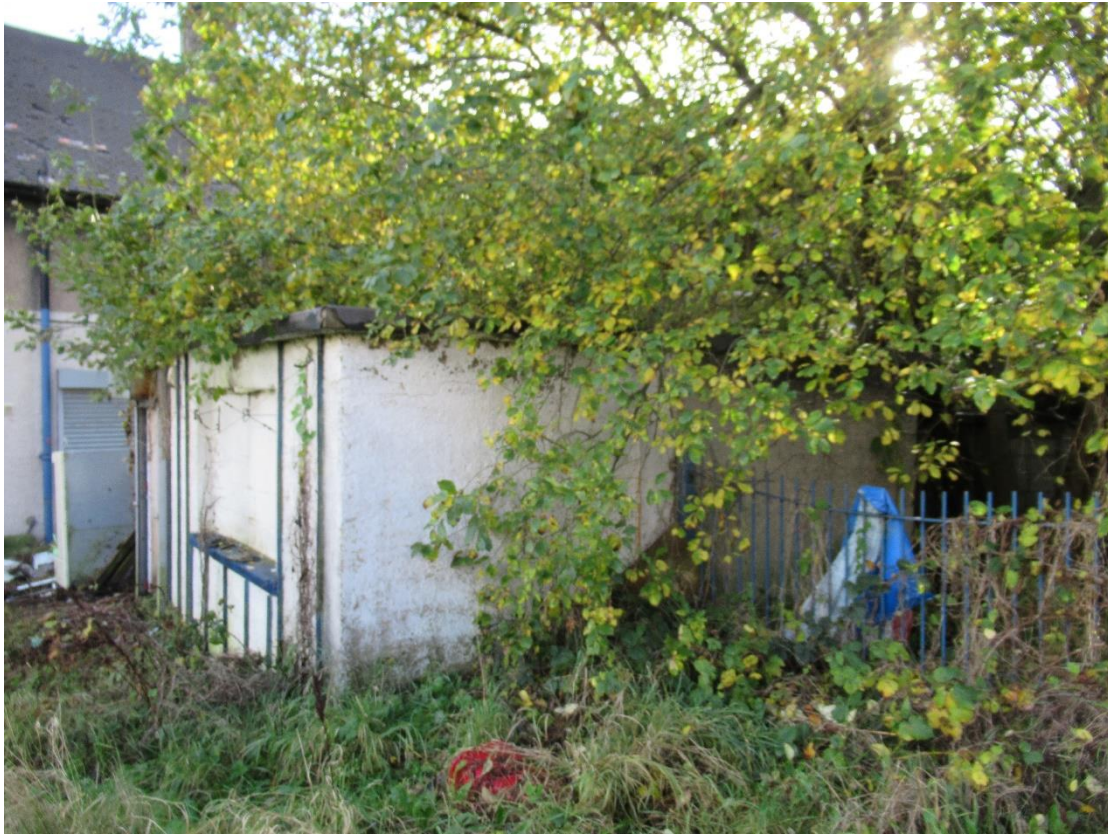
Photograph 27 - External view of northern aspect of Building 2.
