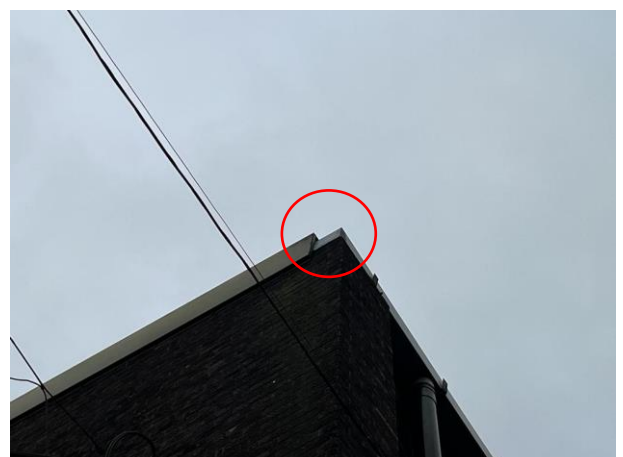
Photo 6: Lifted flashing on the north-eastern corner of the building.
