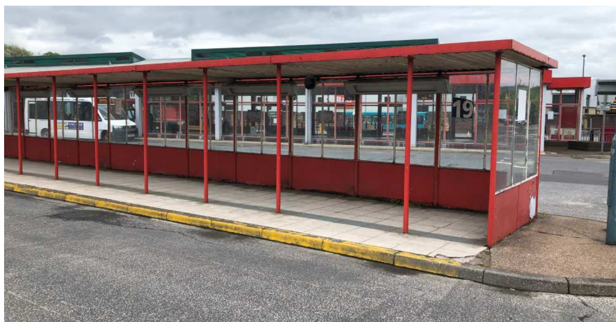
Figure 12 Existing Unused External Coach Stand
