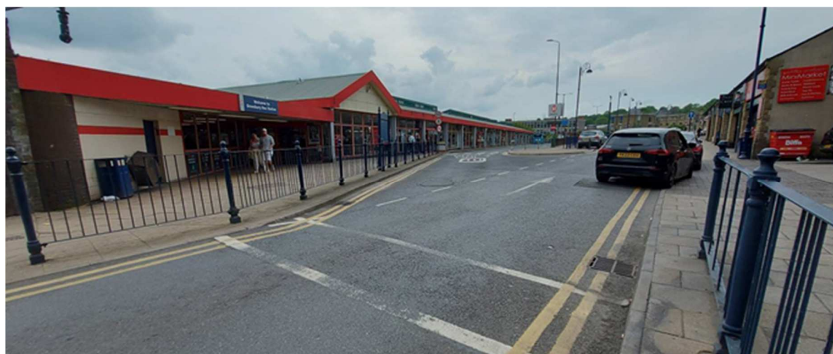
Figure 28 Viewpoint 6 – View up South Street to Dewsbury Bus Station
