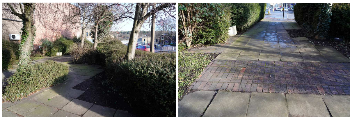
Figure 20 Overgrown Landscaping and Poor-Quality Paving Opposite Dewsbury Minster
