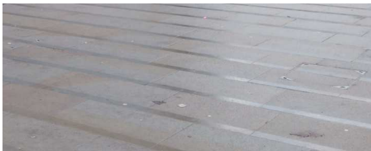
Figure 62 Image of typical paving pattern. Diamond Cut and Shot Blasted Yorkstone Paving.
