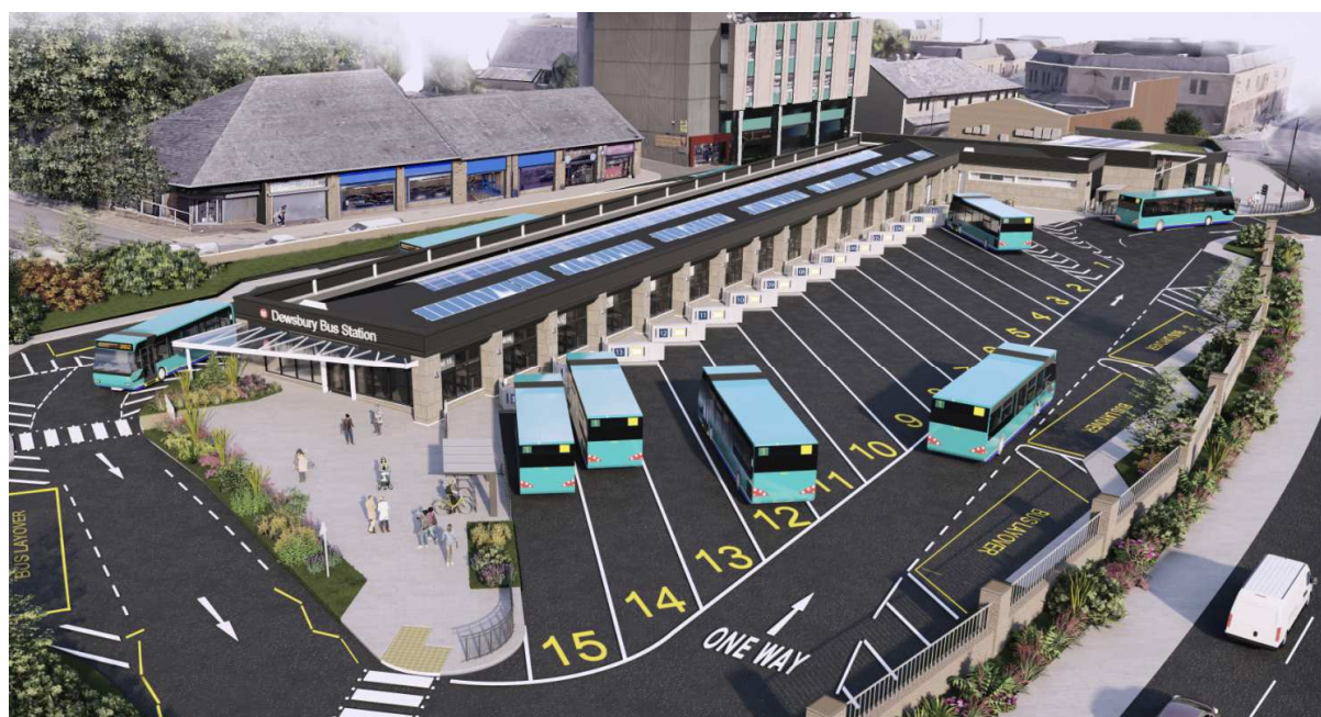
Figure 81 Aerial View showing new photovoltaic Panels
