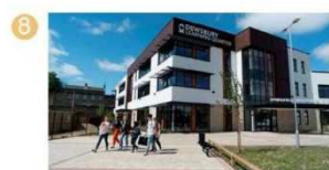
Opened in 2018, a state-of-the-art Centre delivered by the West Yorkshire Combined Authority, through Leeds City Region Growth Deal.
