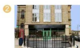
Benefiting from a Townscape Heritage Initiative (THI), the Northgate House Refurbishment consists with new shopfronts, a new flat roof and new windows.
