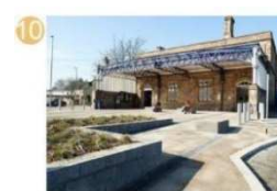
The train station saw a £1.2million facelift in 2019, thereby creating a more attractive entrance to Dewsbury for visitors and commuters.
