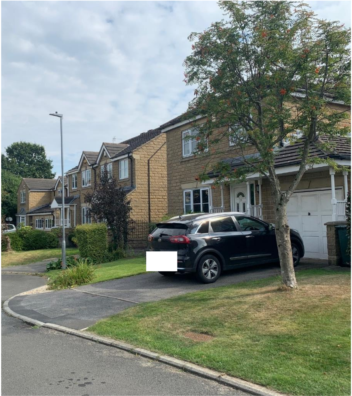
Detached/ semi-detached two storey stone dwellings to Ventnor Close
