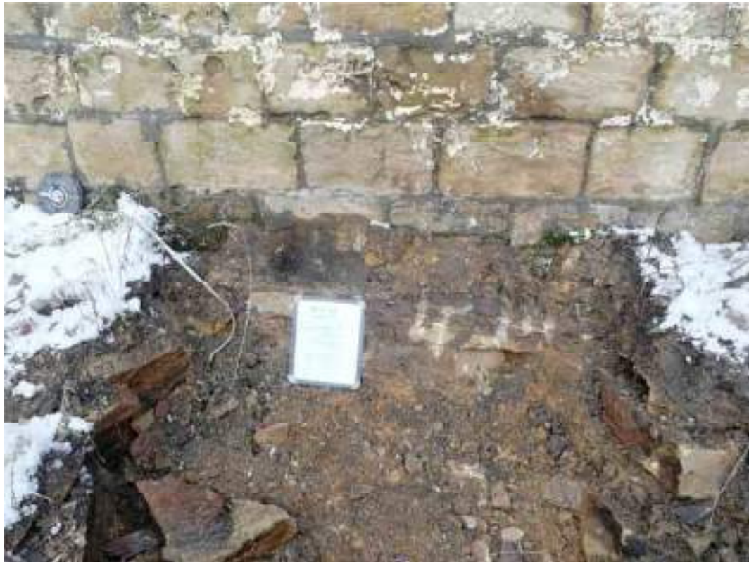
Photograph 3: Exposed foundation of the sandstone retaining wall in TP6.
