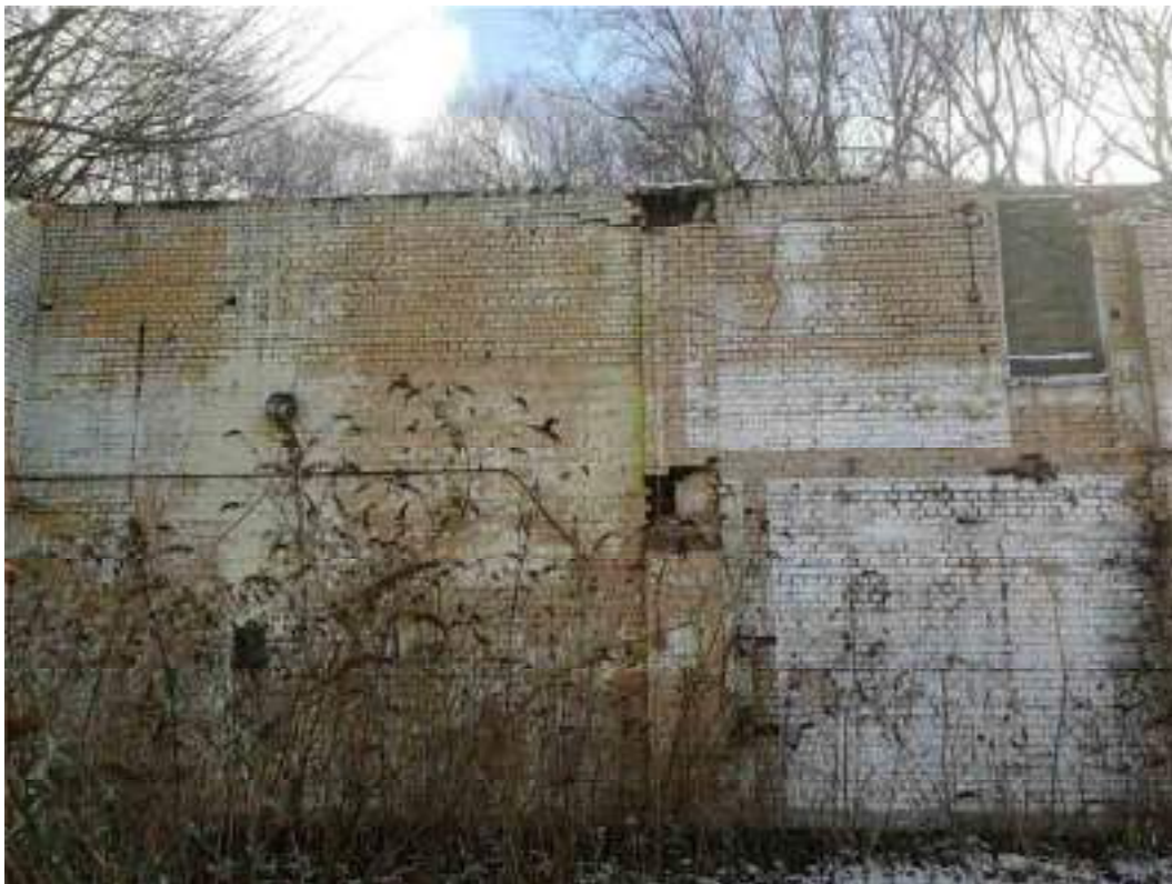
Photograph 19: Retaining wall along eastern boundary of Area B.
