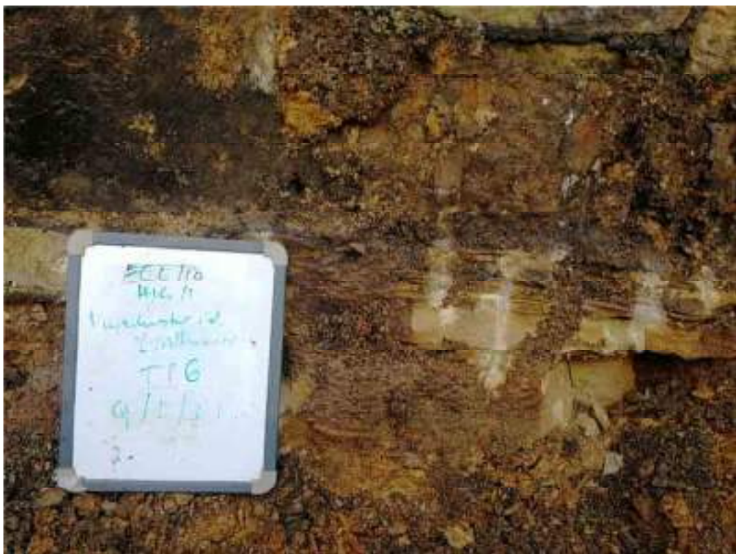
Photograph 4: Close-up of exposed foundation in TP6
