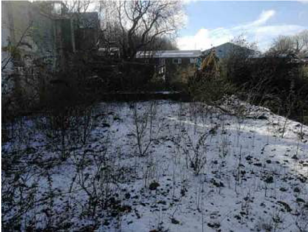
Photograph 20: At the top of the sandstone retaining wall in photograph 1, facing southwest.
