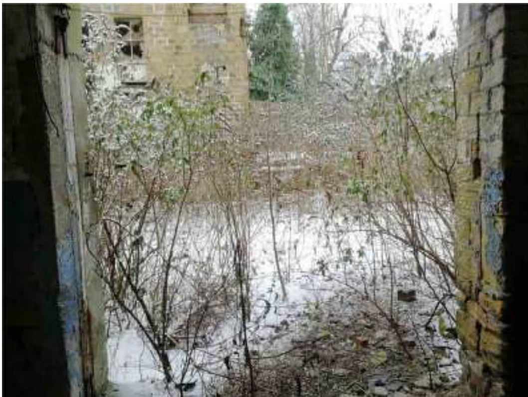
Photograph 17: View from opening in larger building looking towards the smaller building.
