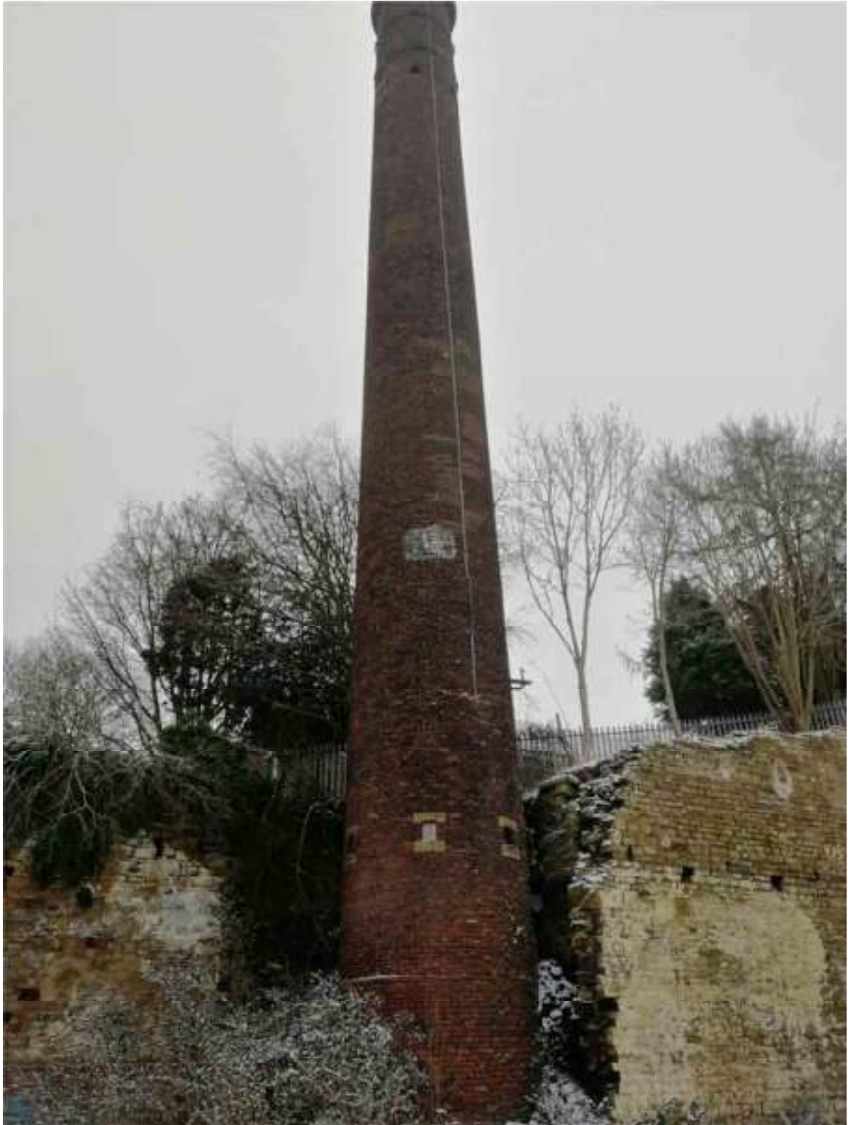
Photograph 13: Chimney at northern end of Area A.
