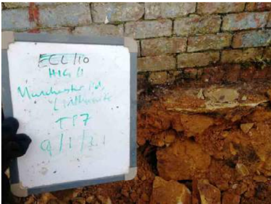
Photograph 9: Close-up of exposed foundations in TP7
