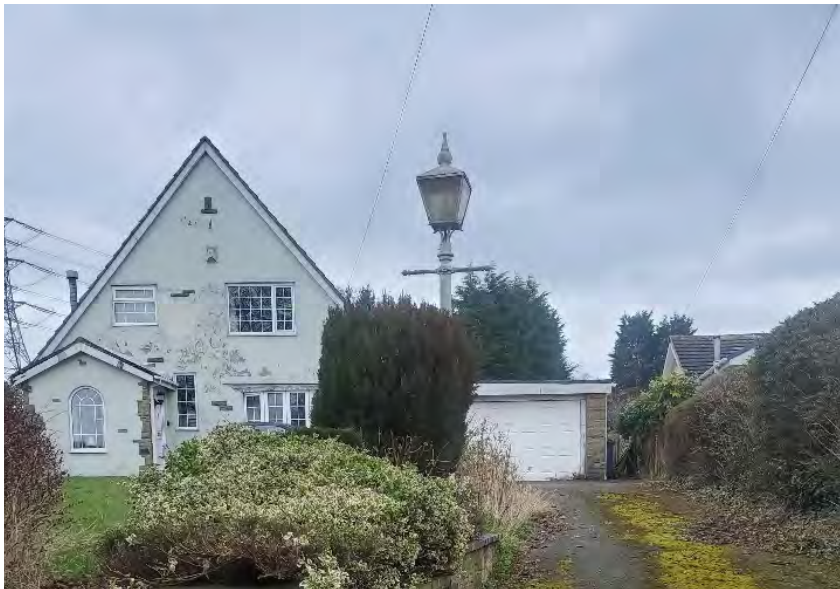
FRONT ELEVATION FROM SHARED ACCESS ROAD
