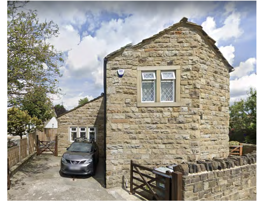
207 Drub Lane - traditional older property
