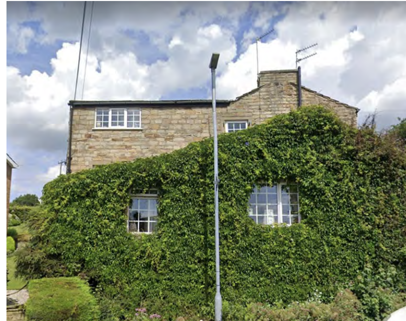
185 Drub Lane - traditional older property
