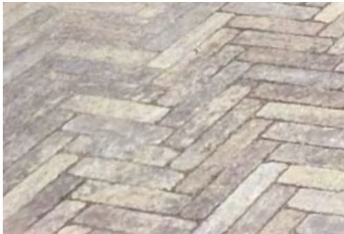
Stone coloured paving to patio, roof terrace and paths
