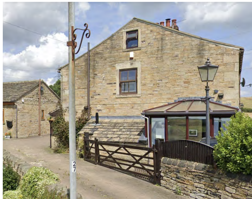
227 Drub Lane - traditional older property
