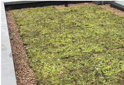
Laid on tray, green roof beyond roof terrace.
