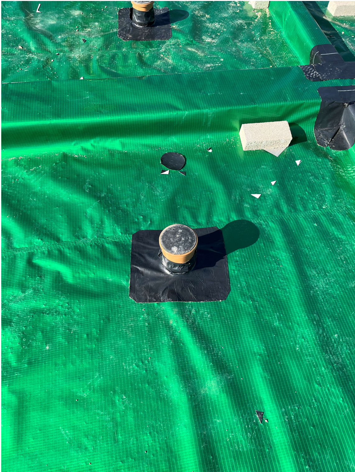
Plot 9 & 10 – Tophat & membrane layout with jointing
