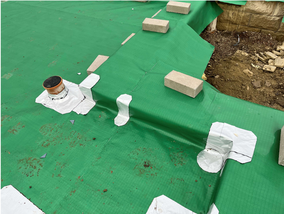
Plot 11 – Tophat & membrane layout with jointing
