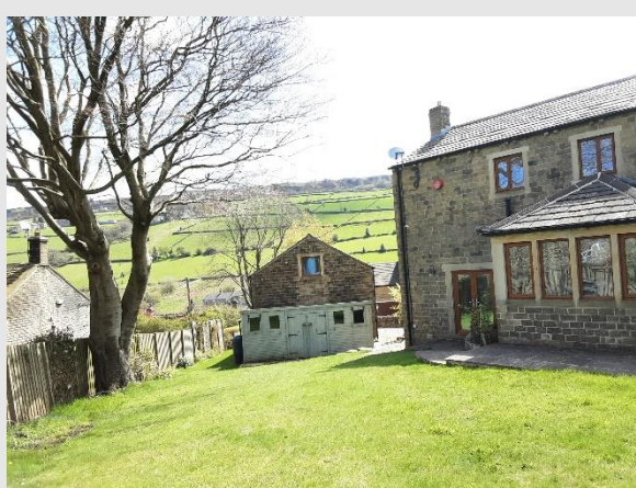
Plate 4: T001 and existing extension
