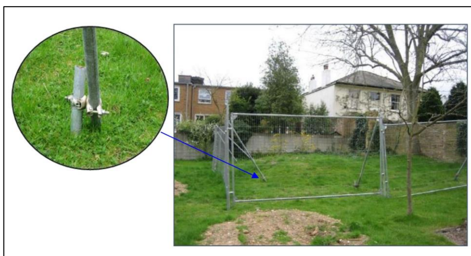
Figure 4.1: Example of mesh welded type barriers in-situ
