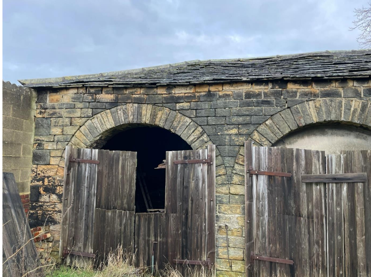
Figure 29 Stone arches to west elevation.
