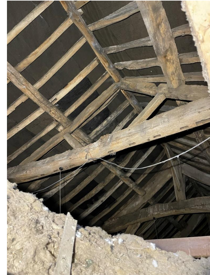
Figure 10 Replacement truss to foreground with typical king post truss with cambered bottom chord to background in main barn.
