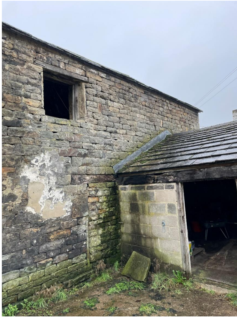
Figure 15 Timber lintels to east elevation.
