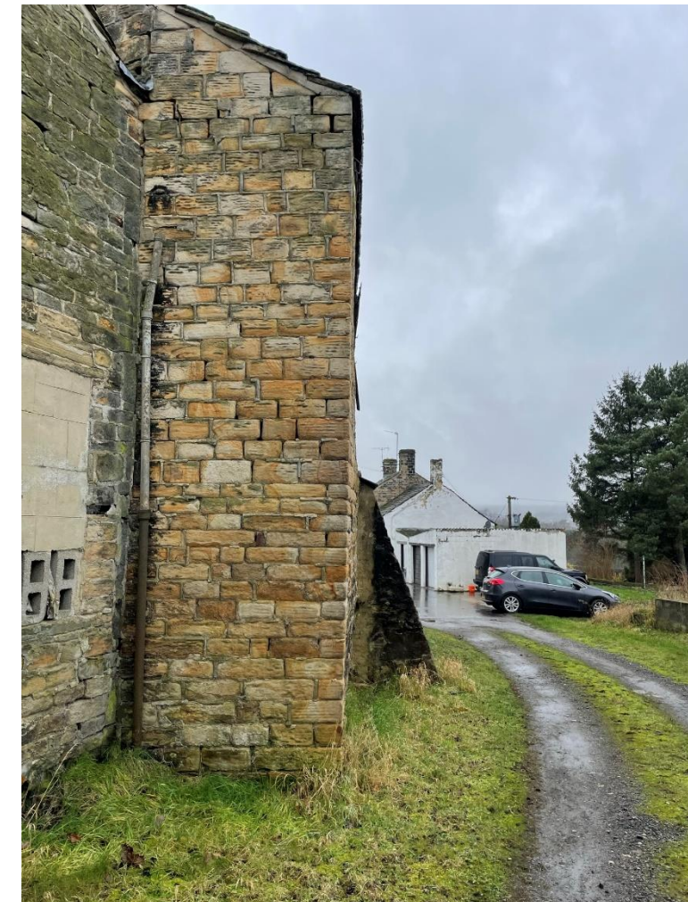
Figure 17 Distortion of north elevation viewed from east.
