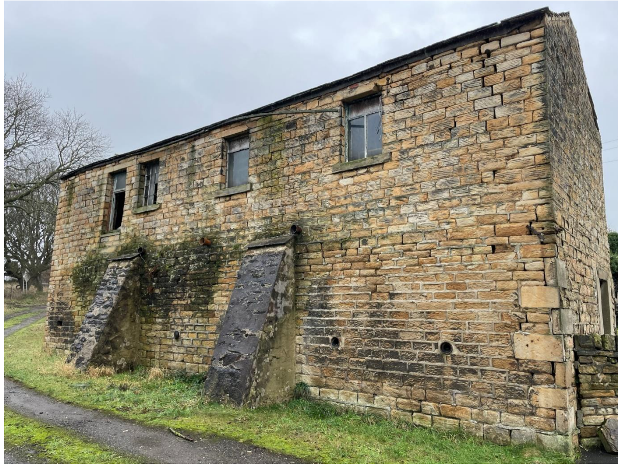
Figure 8 North elevation with stonework buttresses
