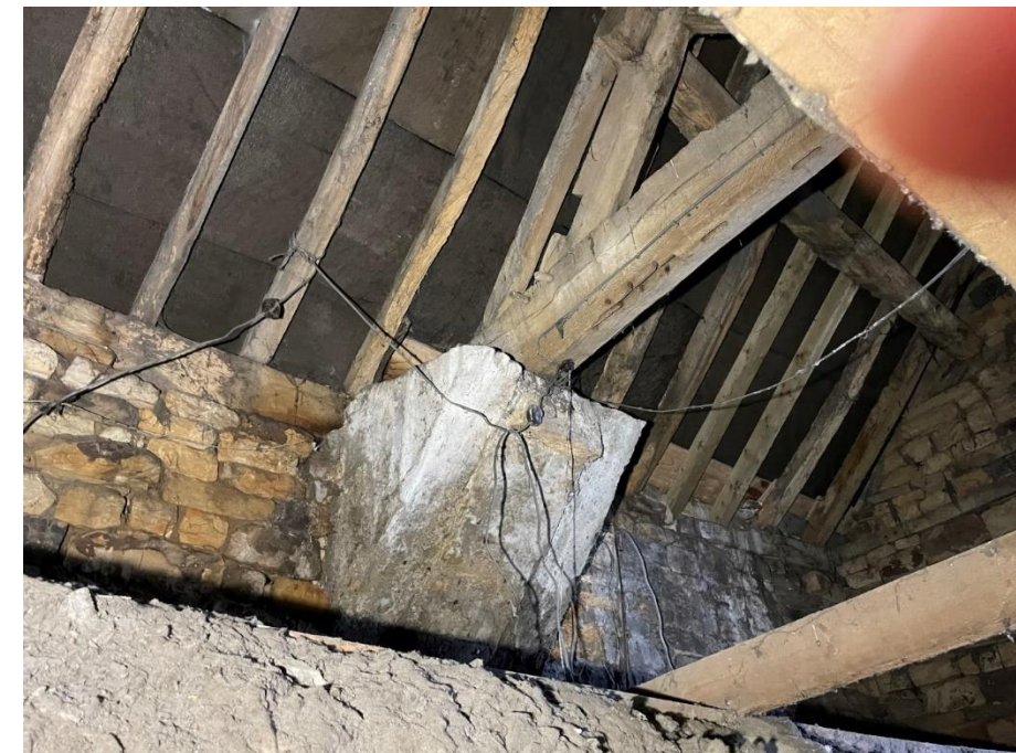
Figure 11 Corbel supporting replacement truss.
