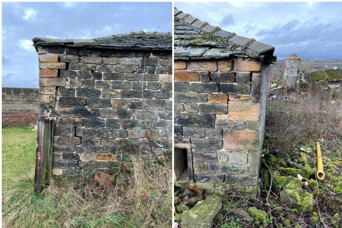
Figure 26 Movement to south elevation (a) West corner (b) East corner.
