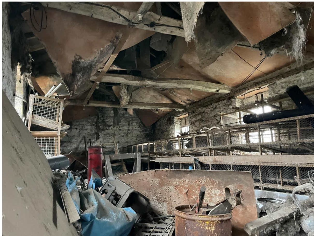
Figure 6 First floor as viewed from doorway at top of steps in south-east corner, with views of queen post trusses.
