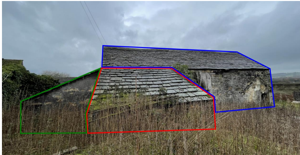
Figure 9 Stone Barn C viewed from east. Blue: Main barn; Red: Single storey to east; Green: Single storey extension to south. Note: brickwork and blockwork extension to west not visible.
