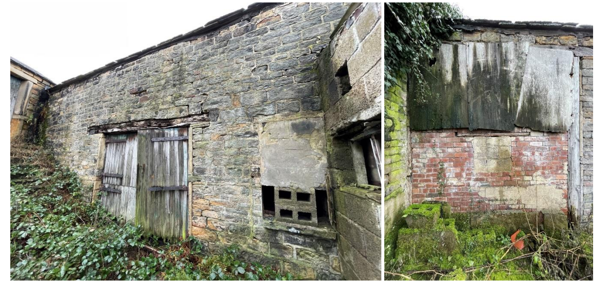
Figure 22 (a) Door opening to west elevation with timber lintel; (b) Large infilled opening to east elevation with timber lintel.
