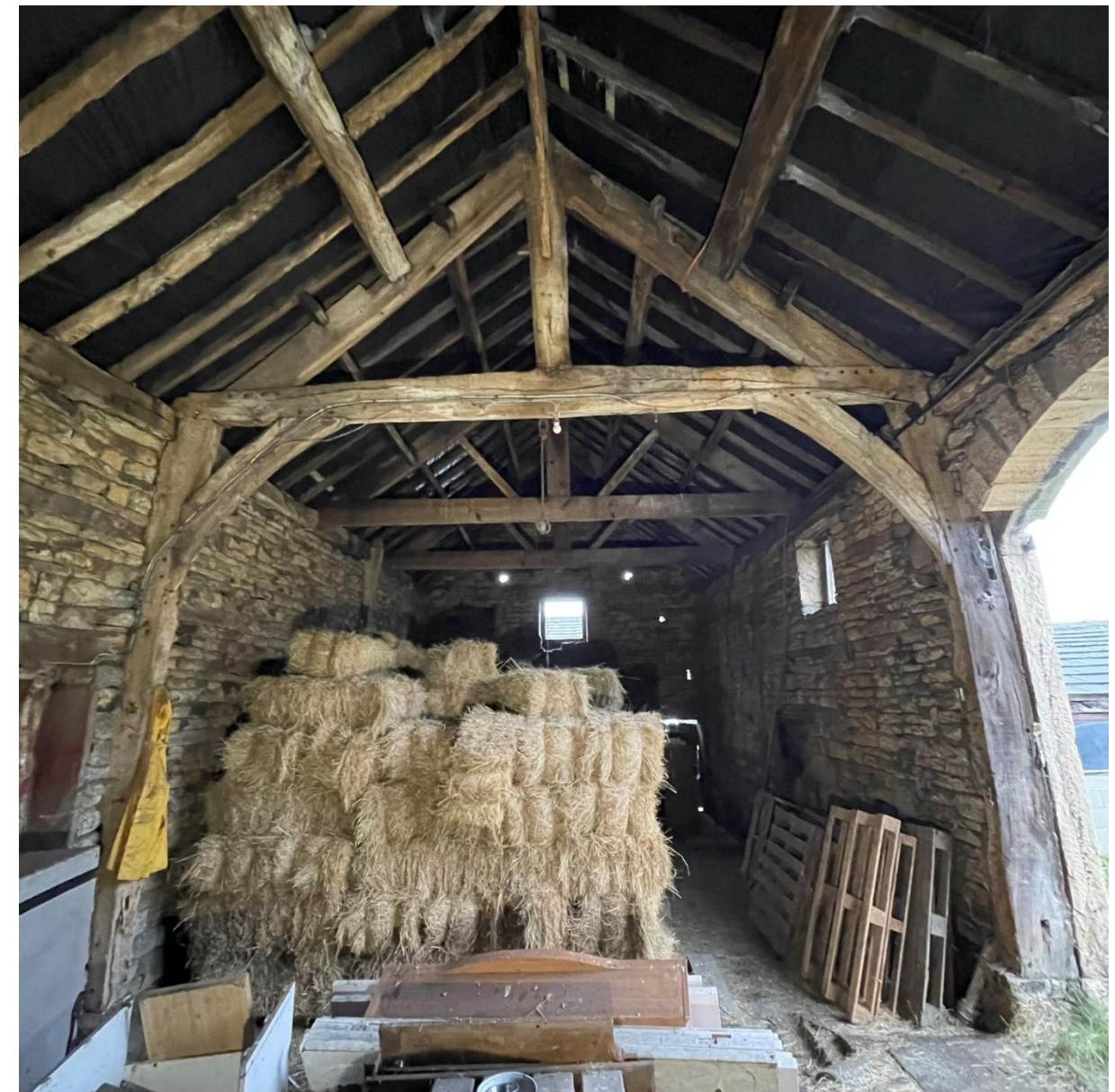
Figure 5 King post truss to foreground on timber posts with bracing and two queen post trusses to background having replaced a single original king post truss (note: timber columns to original king post truss are still present in wall).
