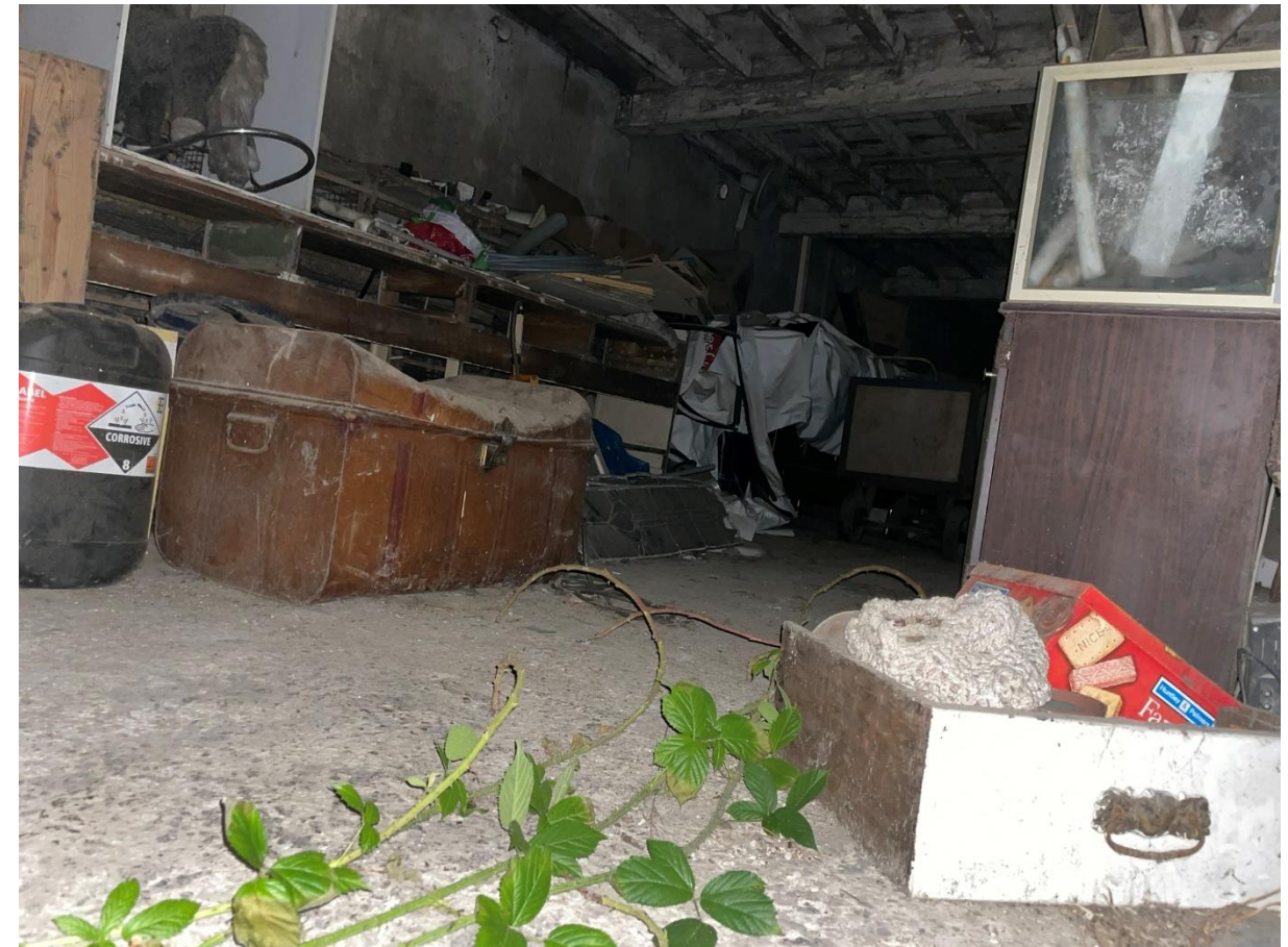
Figure 7 View of ground floor from doorway to west elevation with view of underside of first floor construction.
