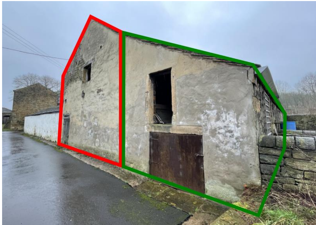
Figure 4 Stone Barn A viewed from north-west. Red: Main barn; Green: Single storey.
