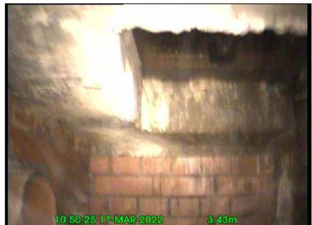
Photo: 4_10A 3.4m, Finish node type, manhole reference number: MH01
