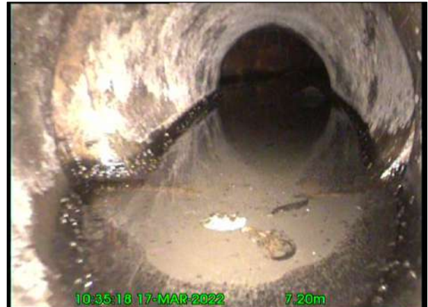
Photo: 1_7A 7.4m, Clear water level, 20% of the vertical dimension
