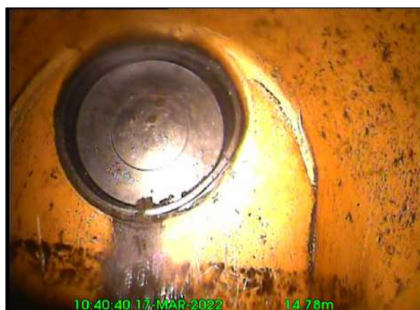
Photo: 2_15A 14.75m, Finish node type, gully reference number: Pipe B
