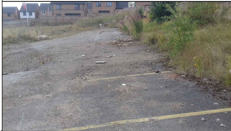
04. Grassed bank and remnant asphalt car park surface
