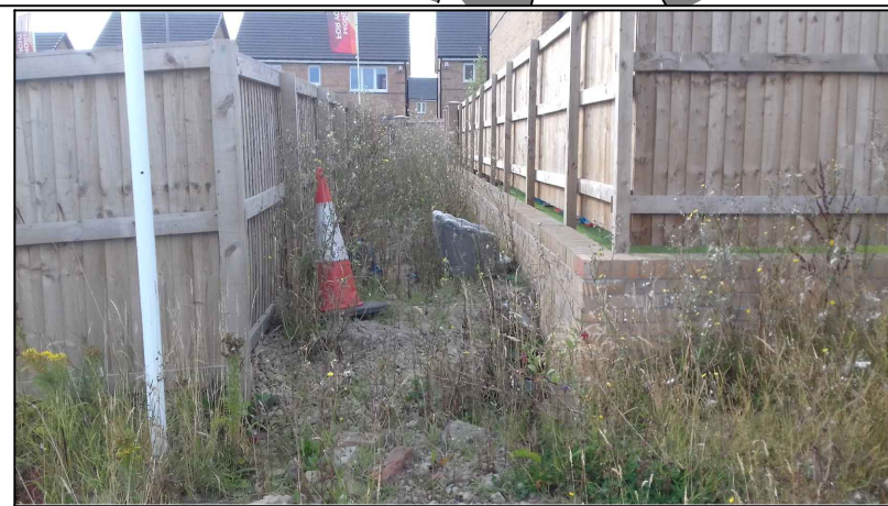
05. Low brick retaining wall to garden adjoining site
