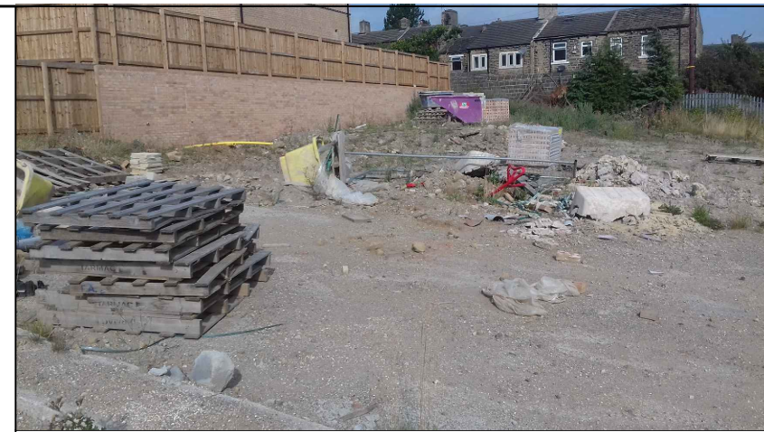
03. Brick retaining wall at site boundary, and builders waste on the site
