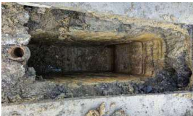
Photo 1 View of pit.
