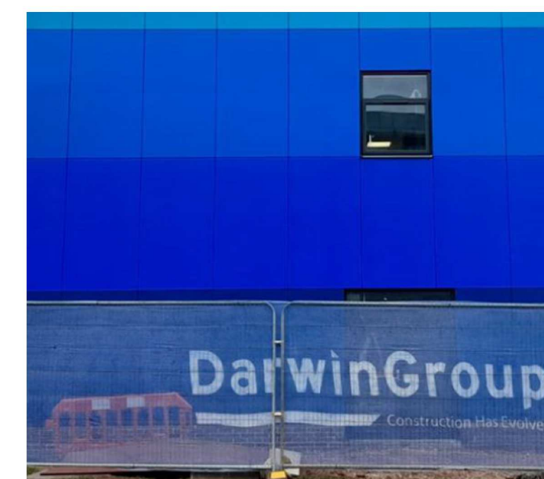
Heras Fencing with Debris netting
