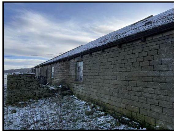
Rear Elevation of Milking Parlour
