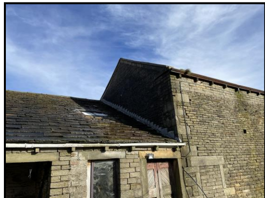
Left Hand Gable of Main Barn
