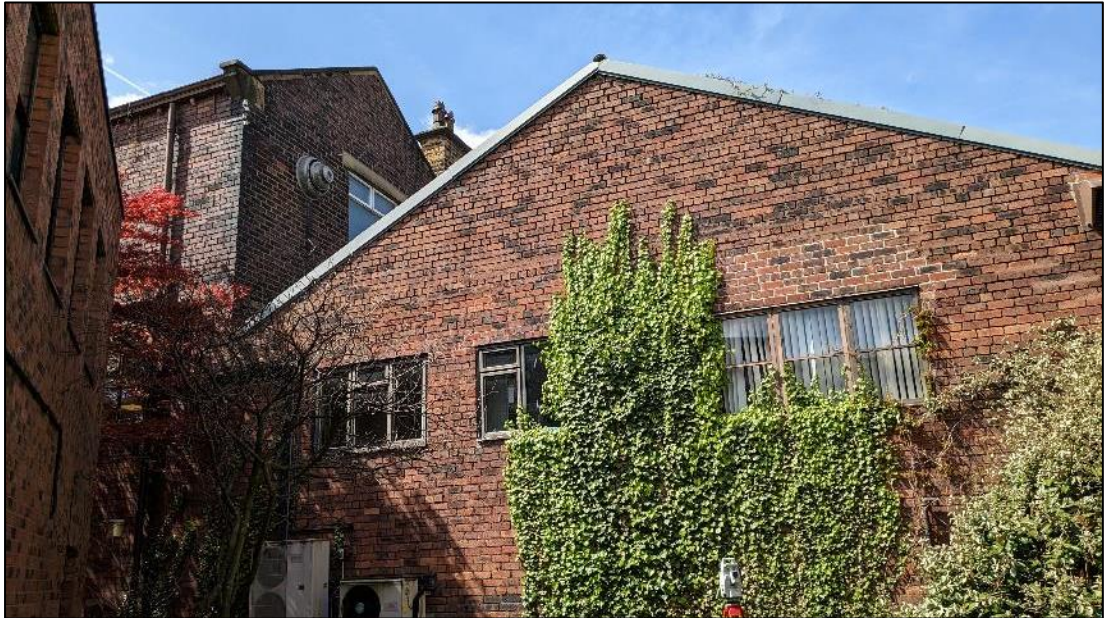
Plate 1. East gable of B1
