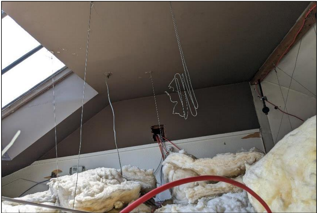
Plate 6. Partly vaulted section of roof, with skylights, in B2
