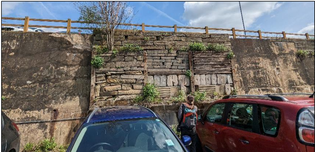
Plate 15. Section of retaining wall built from stacked stone
