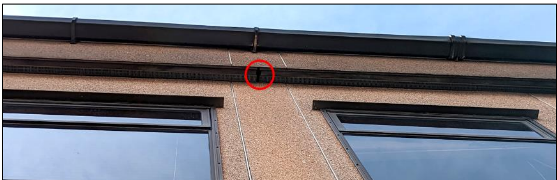
Plate 8. Example space between sections of insect mesh between fascia and wall on B5
