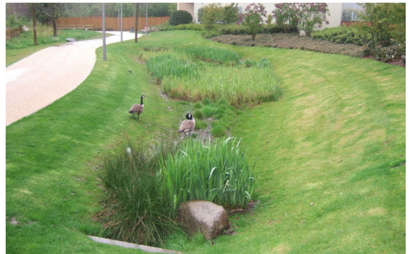
Example of a swale provided by Bright Young Consulting.
