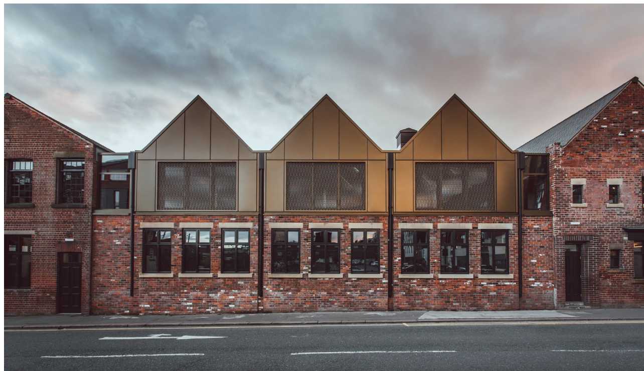
Albert Works, Sheffield (Disused Warehouse Refurbishment by City Estates/ Jaywing/ Cartwright Pickard Architects)
