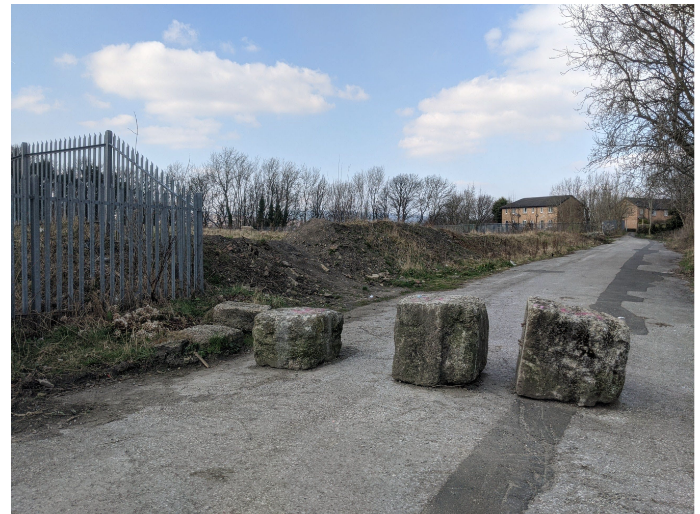
Current view along Hart Street (Photo dated 20 March 2022)
