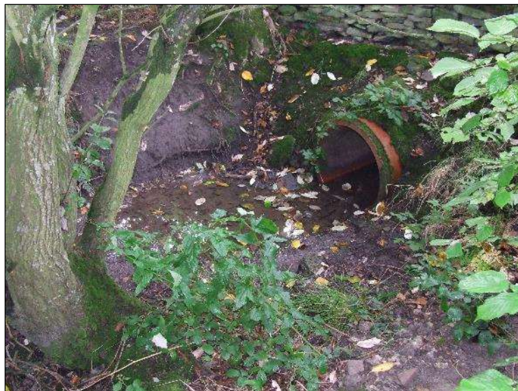
Photo 18: Sampling point SW02 from East Hill Beck. The pipe represents the entrance to a short culverted section of the beck.
