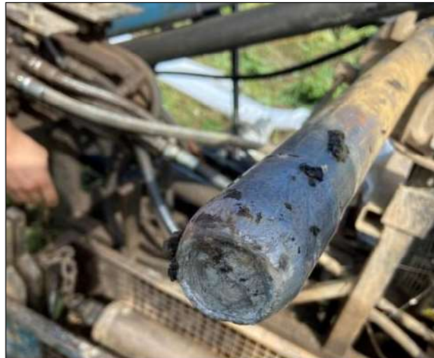
Photo 13: WS04 – Close up of the weathered siltstone at the base of the exploratory hole.
