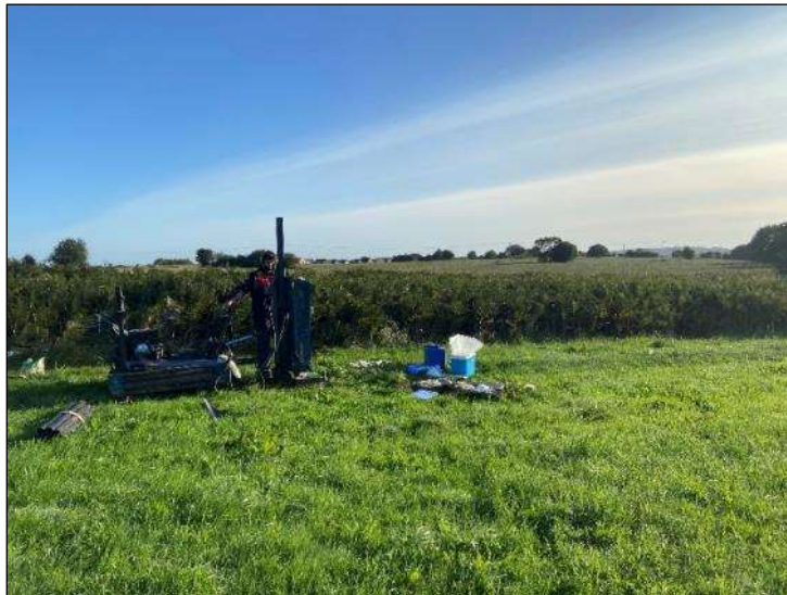
Photo 1: WS01 – Position of the first window sampling location on eastern part of historic landfill.
