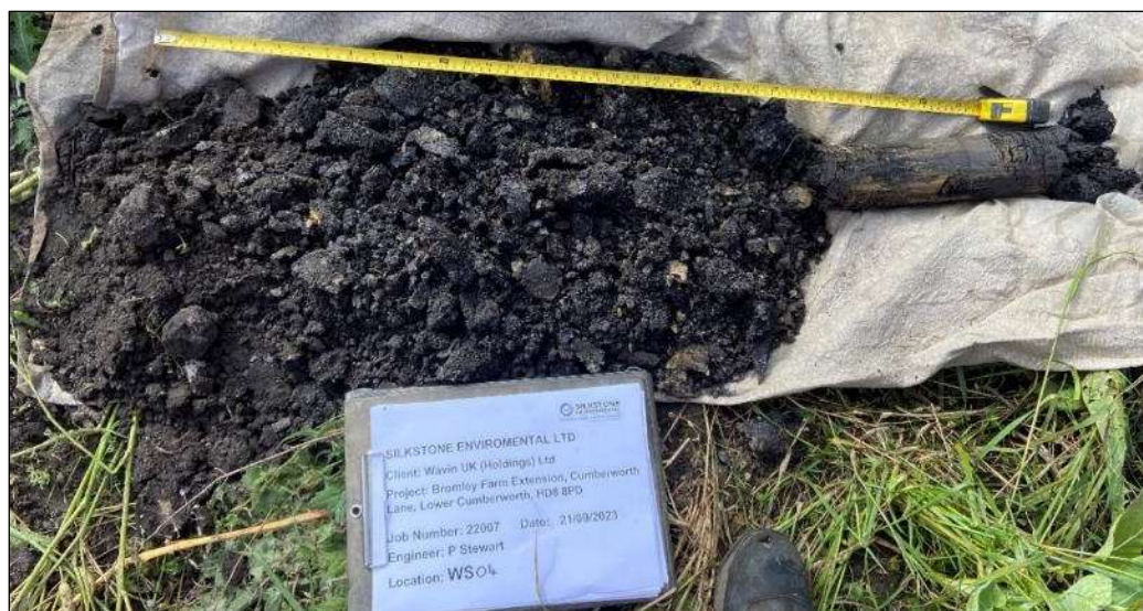
Photo 11: WS04 – Made Ground (Topsoil) arisings from hand dug inspection pit and window sampling (depth progressing from left to right).
